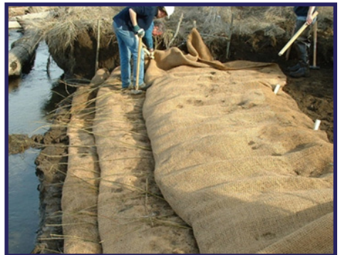
Live staking between lifts with coir blanket.
