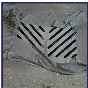
Sediment fence fabric does not filter and causes ponding at the surface.
