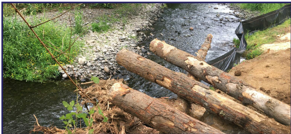
Consider perimeter controls when installing LWD installations.
