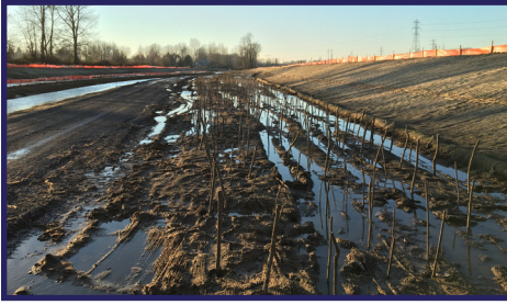
Live staking through jute.
