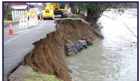
Emergency response from washout to protect public infrastructure and restore the roadway.
