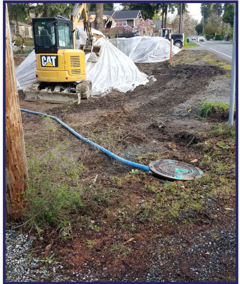
Dewatering to sanitary under an approved permit.
