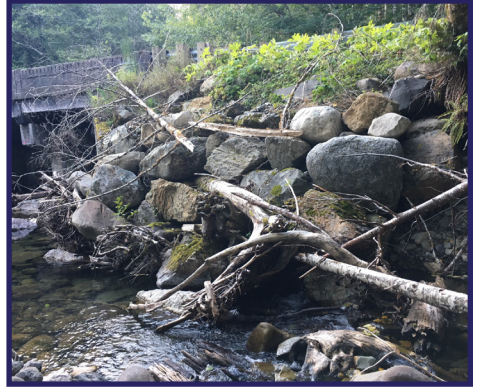
Rock protection at bridge abutment.
