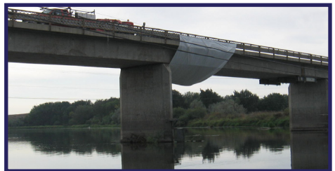
Bridge containment system for painting work.
