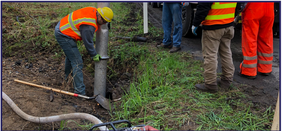
Vactoring a culvert to allow for system flow.
