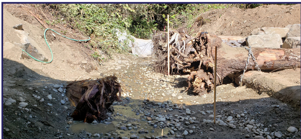
LWD being embedded in bank and anchored with chain and deadman anchors.
