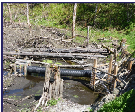
Example of cage system with tube.
