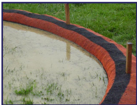
Compost socks allow for three dimensional filtration and can be placed right on the ground.
