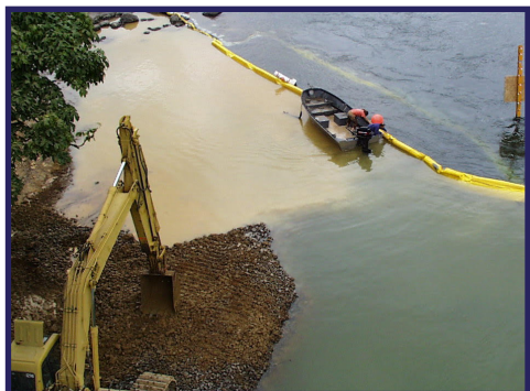
Turbidity curtain is installed outside of flowing water, using multiple curtains to ensure entire job length is encompassed. Sign is installed on opposite bank at water point of entry warning summer water enthusiasts to beware of construction site.
