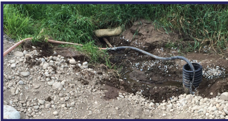
Dewatering from a wellpoint within a maintenance project.
