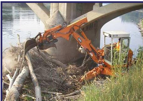
Relocate large woody material (LWM) from bridge pier.
