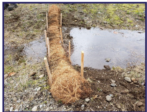
Coir log wattles can be left on site and will biodegrade in 24-48 months.
