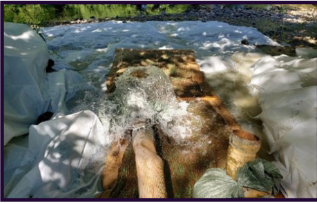
Plastic, silt mat, hose with elbow, sandbags to keep hose stable. Elbow allows extra dissipation through pushing water into air.
