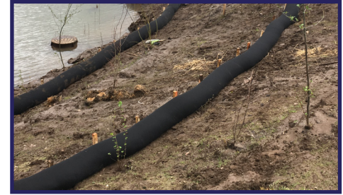
Slope checks help retain soil for plantings in tidally influenced areas.
