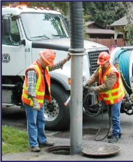
Dewatering an enclosed drainage system.
