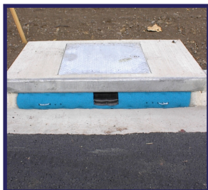
Recessed curb inlet dam to remove coarse material prior to filter.
