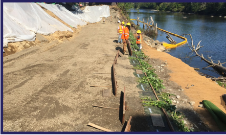
Planting, live potted dogwood, on streambank geogrid multi-layer wrap repair.
