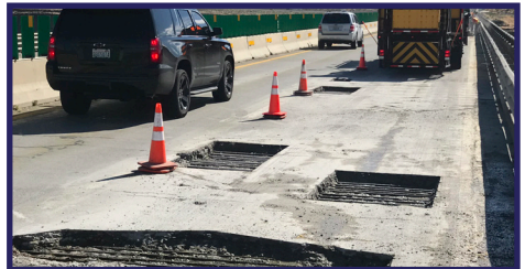
Contain and dispose of concrete material during bridge deck repair.
