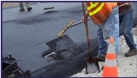
Protect drain inlets when repaving.
