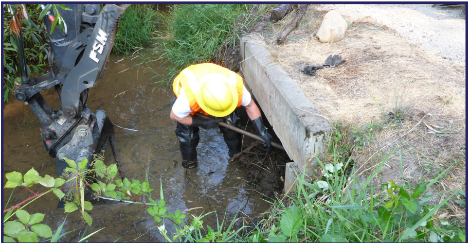
Cleaning beaver debris from a box culvert. Follow safety precautions.
