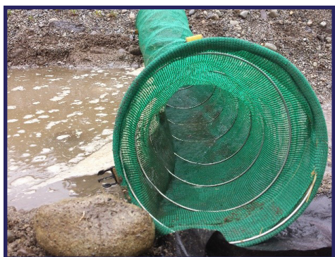
Spring berms are six feet wide and can be clipped together.
