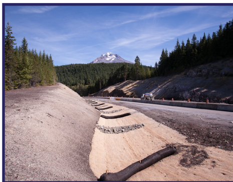
Combination of check dams can achieve better results.
