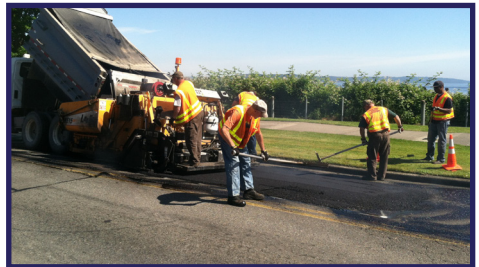
Conduct overlays during dry weather.
