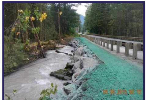
Roadside streambank erosion repair.
