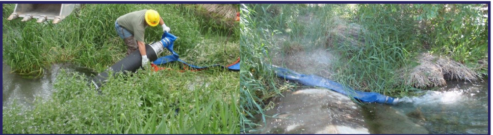
Dewatering a detention pond using culvert plug to bypass water.
