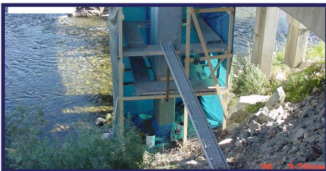
Install containment to prevent material from falling into sensitive areas.
