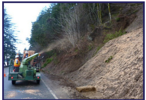
Make sure to apply over 90% coverage when utilize straw mulch.
