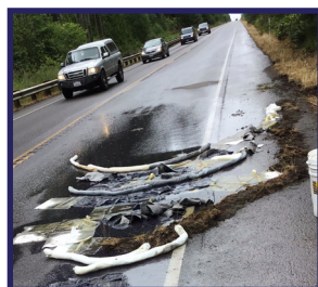
Protect stormwater infrastructure using sorbents and earthen berms.
