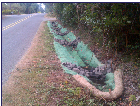
Ditch lining and check dams.
