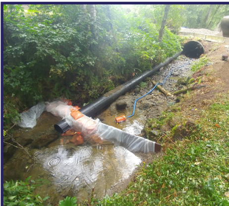
Gravity bypass with steel plate cofferdam.
