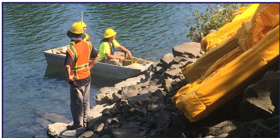
Preparing for installation – land spotter, water craft, wearing PPE including life jackets.
