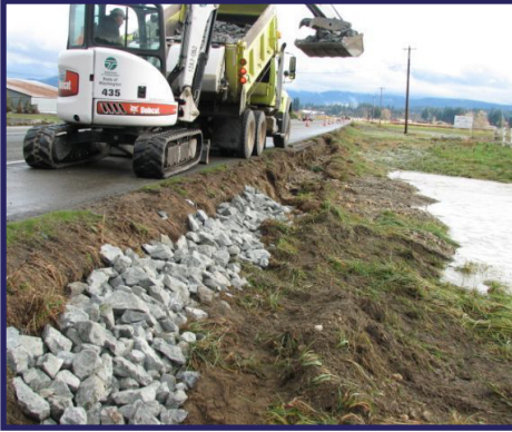
Repairing shoulder erosion with rock.
