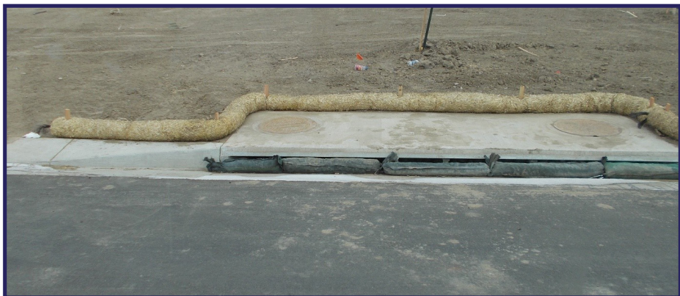
Gravel sock as prefilter in high flow environments.
