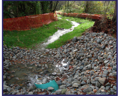
Rock outlet energy dissipater.
