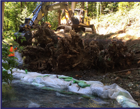
Sand bag cofferdam providing a dewatered work space.
