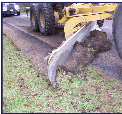
Shoulder grading to ensure sheet flow of road runoff and leave a vegetated strip.
