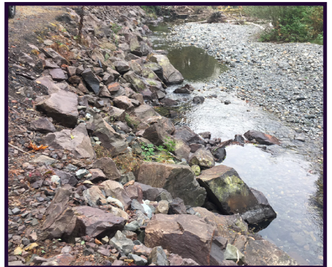
Rock and large woody material (LWM) used for roadside streambank repair.
