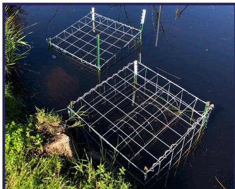
Example of culvert cage set in open water environment. Cages may be designed with hinged access for easy cleaning.
