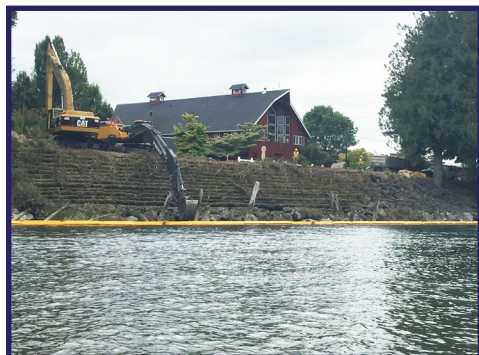
Turbidity curtain is installed outside of flowing water, using multiple curtains to ensure entire job length is encompassed. Sign is installed on opposite bank at water point of entry warning summer water enthusiasts to beware of construction site.
