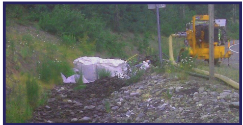
Dewatering a worksite with a pump to bypass flows and work in dry conditions.
