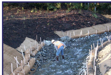
Installing streambed gravel.
