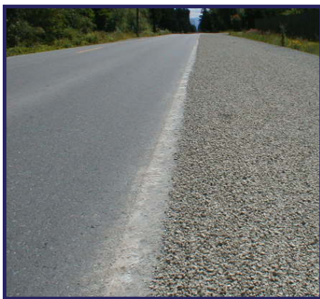
Compact gravel shoulder to prevent erosion and allow for vehicle pull off.
