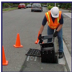
Inlet filter with additional sorbent media for sensitive maintenance project.
