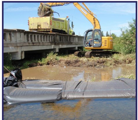
Sediment cleanout from bridge using Aqua-barrier® cofferdam.
