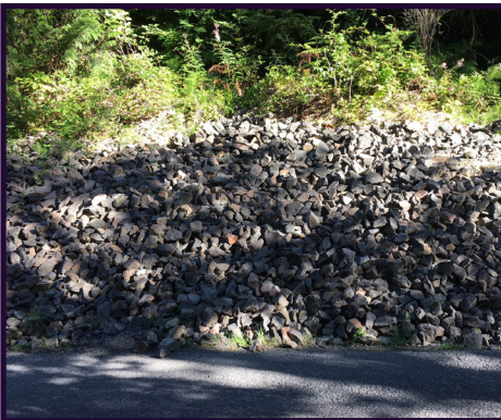
Rock to stabilize roadside slope.
