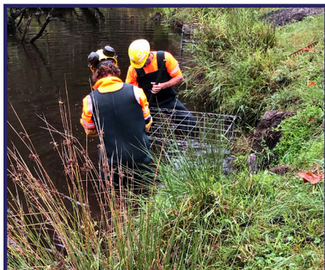
Installation of the culvert cage.
