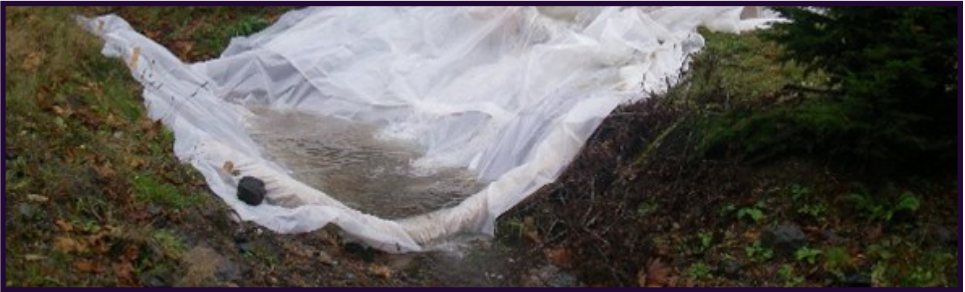
Straw bales and wattles covered in plastic to create velocity reduction and dispersal of water.
