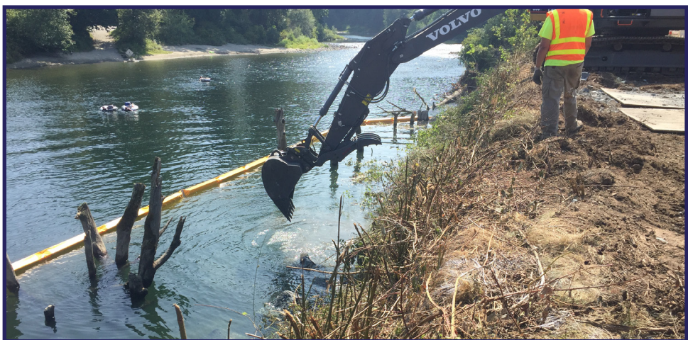
Turbidity curtain is installed outside of flowing water, using multiple curtains to ensure entire job length is encompassed. Sign is installed on opposite bank at water point of entry warning summer water enthusiasts to beware of construction site.
