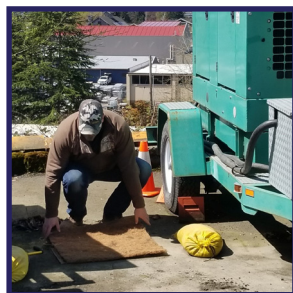
Blocksom™ grate cover with filter underneath.
