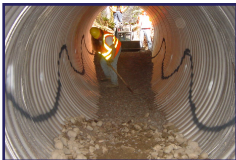
Installing streambed gravel.
