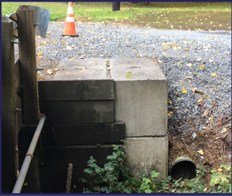
Ecology block to protect bridge abutment.
