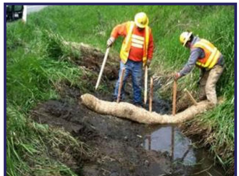
Roadside ditch cleanout and installation of straw wattle checkdam.
