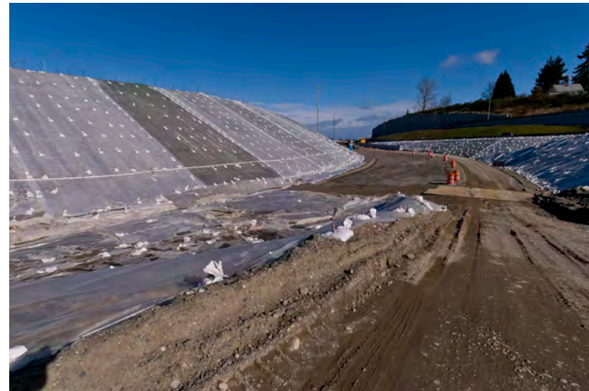
Figure 4. Plastic is used during the construction process to prevent erosion.
