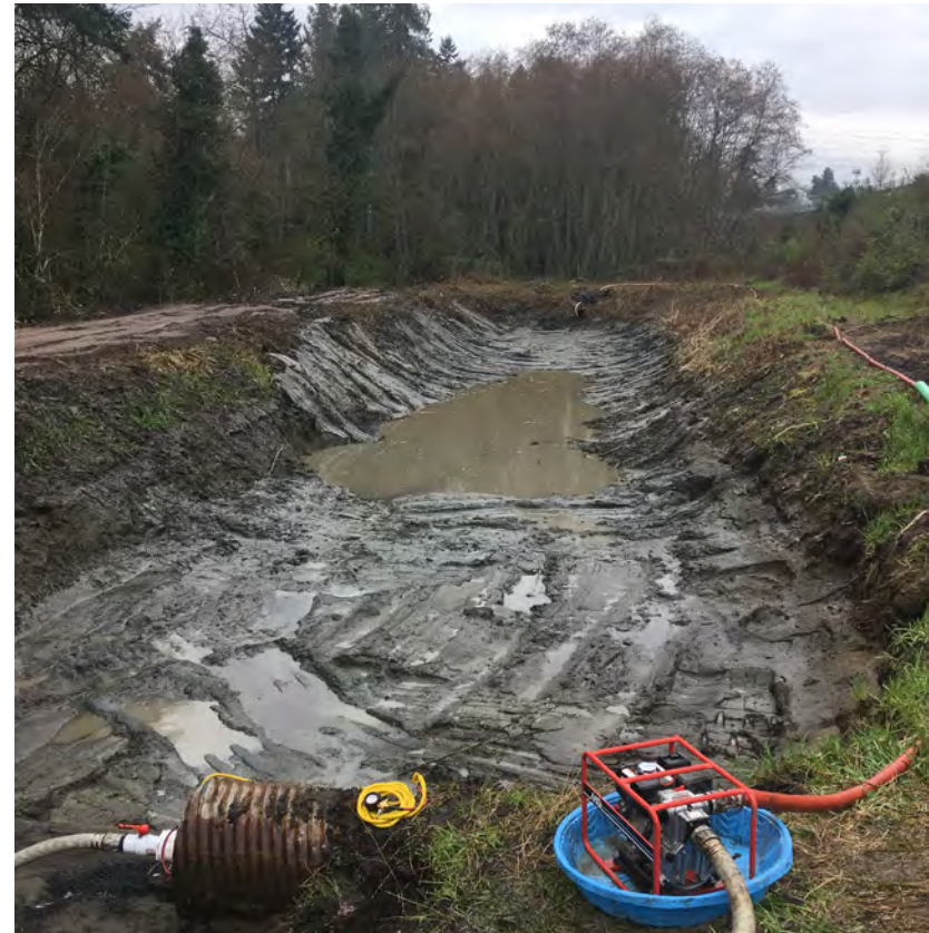
Figure 6. A southwest region pond after sediment removal during phase 2 of the project. Phase 1 and 2 focused on sediment removal. Phase 3 involved retrofitting a berm to divide the pond into 2 cells to help with future maintenance needs and BMP performance.
