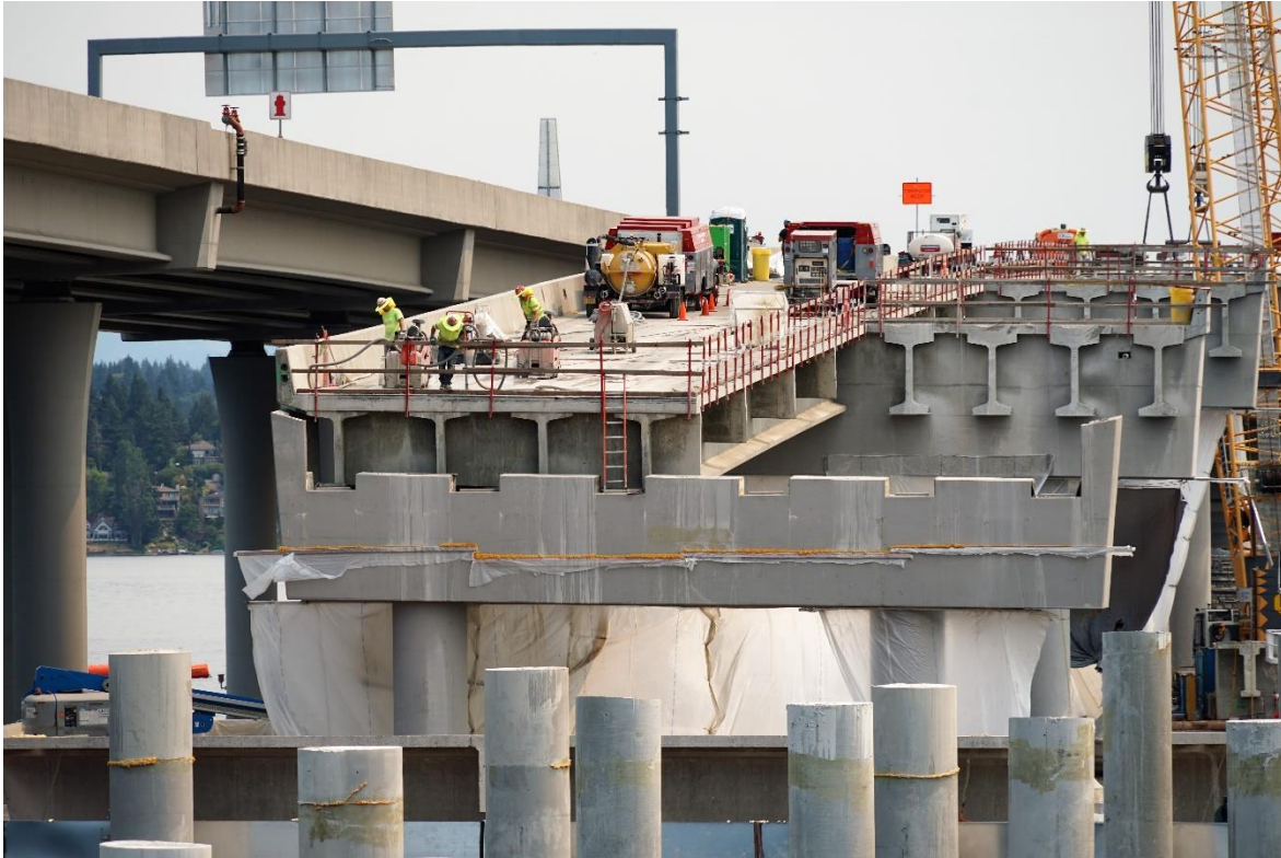
Removing deck spans and girders from the eastern edge of the project.
