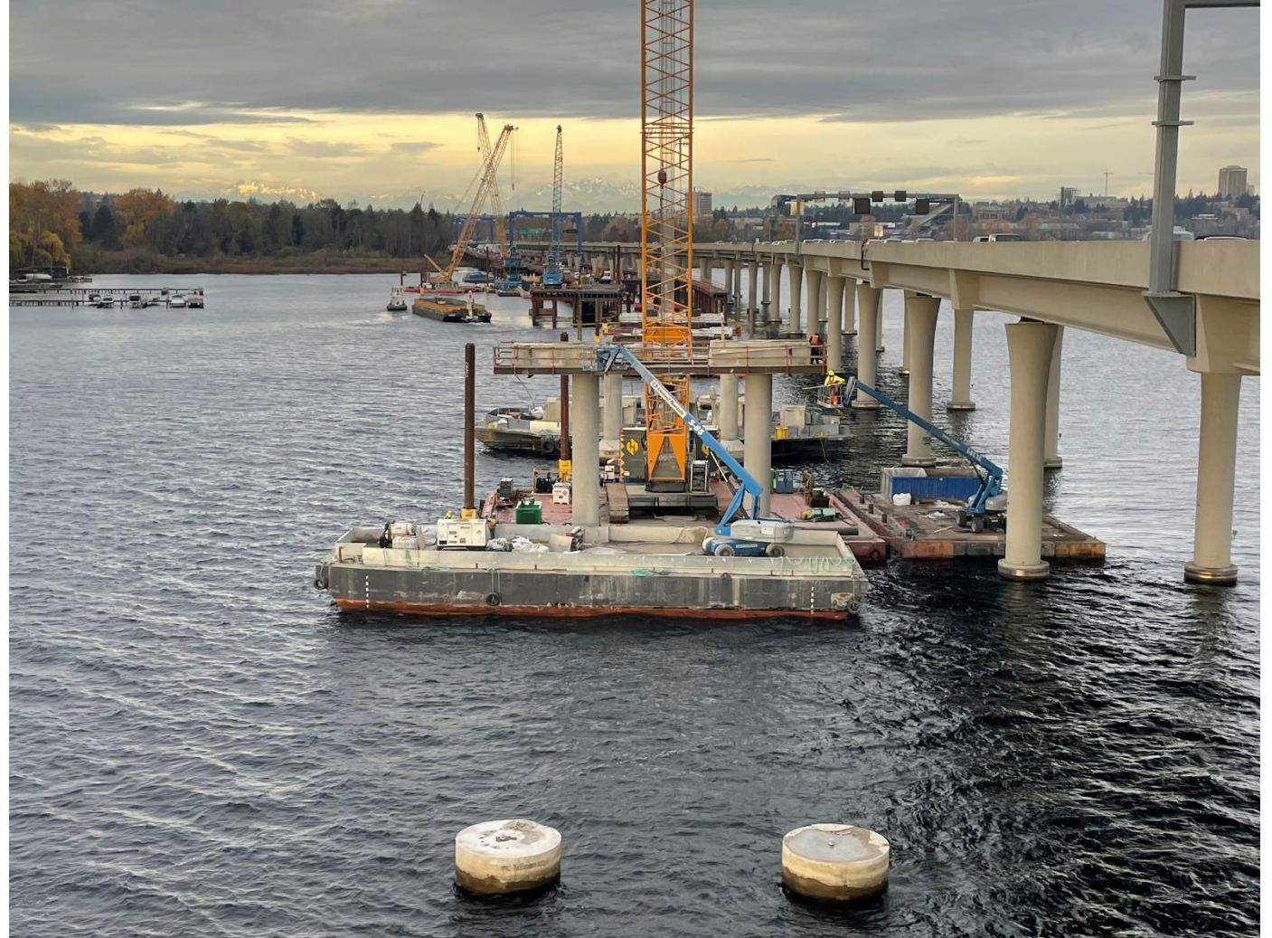
Demolition work on the eastbound SR 520 bridge.
