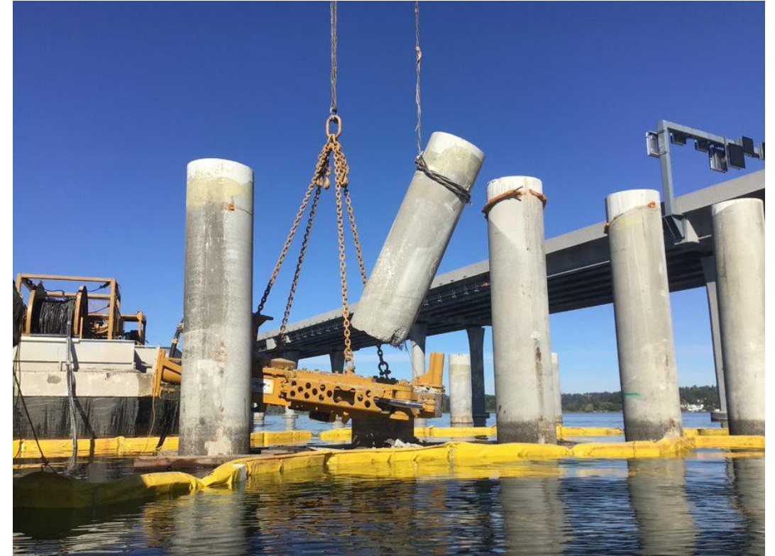
Using equipment hanging from cranes, crews shear the old bridge columns below the lakebed.
