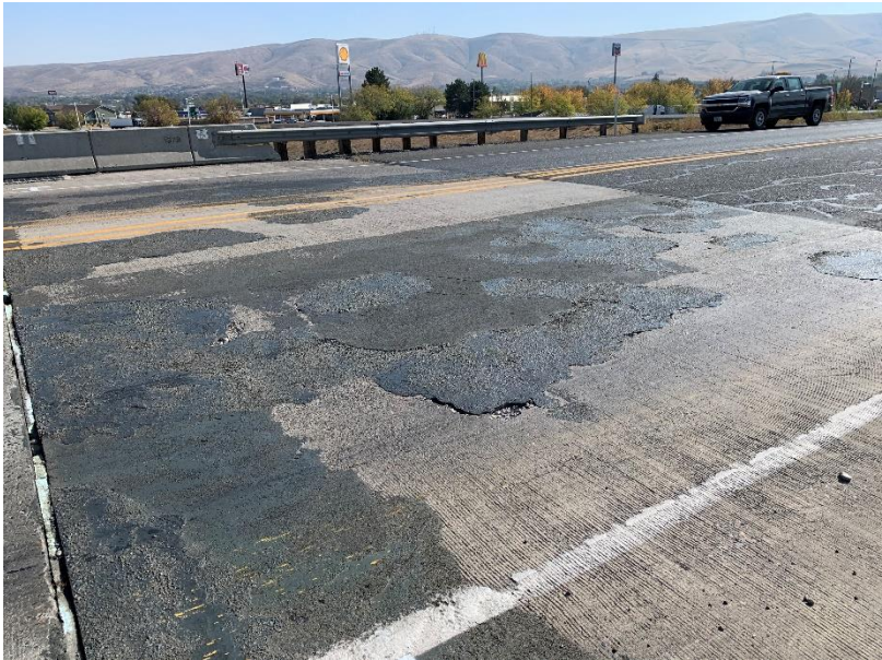
Severe deterioration on a bridge approach at the I-82/Gap Rd interchange in Prosser. Nearly all ramp preservation needs are currently unfunded. Interchanges currently in fair condition (minor cracking and patching) will look like this in ten years. Those currently in this condition will see failed bridge crossings and pavements in need of reconstruction.
