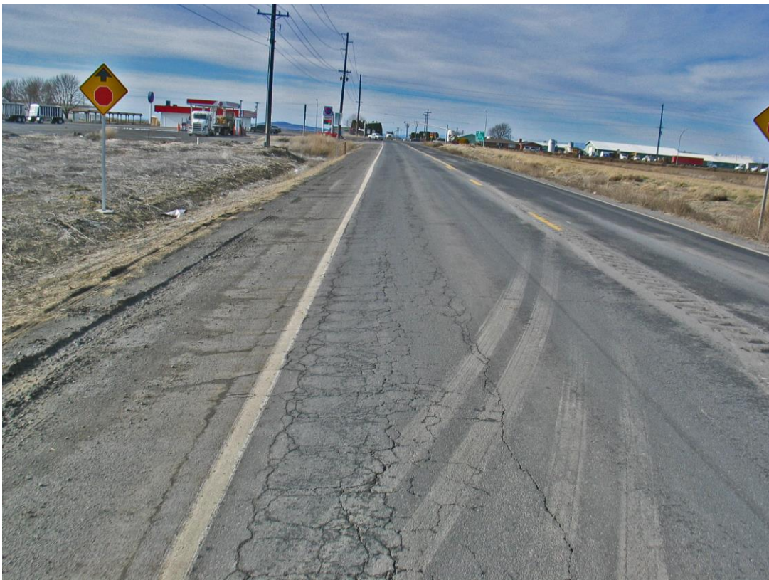
State Route 170 pavement is severely cracked, rutted and rough. Road surface is very rough to traveling public and impacts agricultural hauling.
