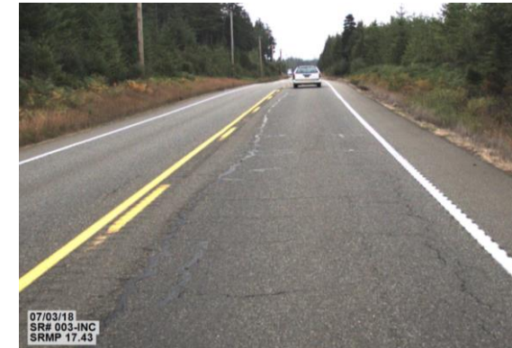
Severe cracking on State Route 3. The surface cracking is widening and rapidly expanding. This will cause the pavement to deteriorate more quickly and result in significantly increase pavement repair costs at the time of the next resurfacing project.
