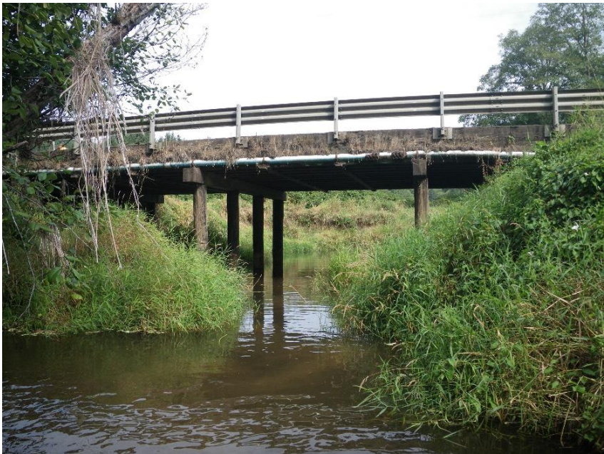
The Hull Creek bridge on State Route 4 was built in 1934. It is a timber bridge that needs to be replaced.
