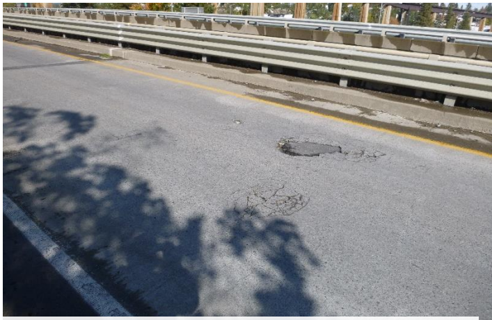
Cracking and patching on the US 195 bridge over I-90. The deck will need to be resurfaced in the next few years.
