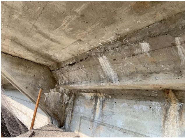
The Palouse River Bridge on US 195 in Colfax has deck deterioration and cracks and the sub-structure (shown). This bridge was built in 1931 and is due for replacement.
