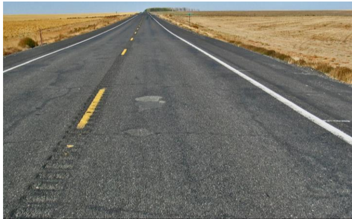
Pavement is rough, rutted and deteriorated. To restore structure, heavier rehabilitation like Cold-In-Place recycling is needed.
