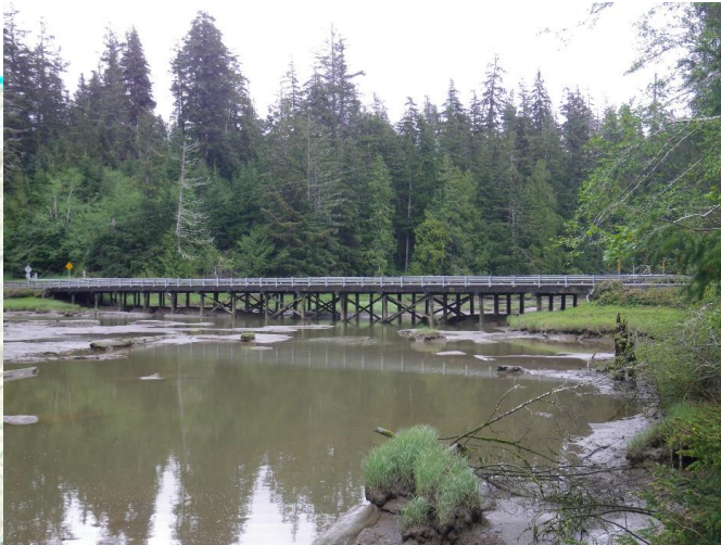
The Teal Slough bridge on US 101 is a timber structure built in 1934. It needs to be replaced.
