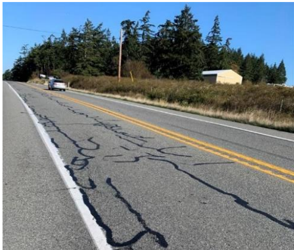
Last paved 20 years ago, the pavement is distressed and deteriorated south of Oak Harbor. Crack sealing has been applied.
