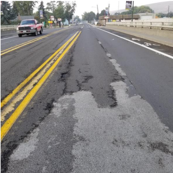
US 12 in Dayton pavement deterioration including rutting, longitudinal cracking and multiple patches.
