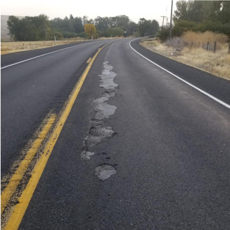
Potholes and delamination on US 12 southeast of Dayton. This section is in need of a chip seal now for optimal, cost-effective preservation, and to prevent it from further deterioration over the next ten years.
