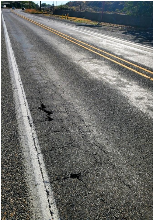
Severe alligator cracking and spalling on SR 224 in West Richland.
