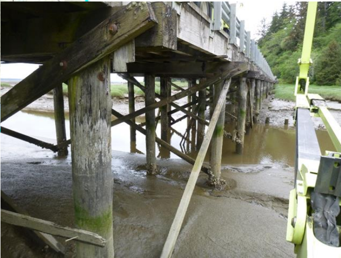
The Greenhead Slough bridge on US 101 is a timber structure built in 1934. It is in poor condition and needs to be replaced.
