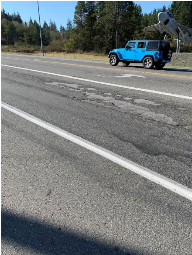
Last paved around 2000, this section of pavement on State Route 20 north of Oak Harbor shows distress and deterioration in varying degrees of severity. Maintenance crews have applied crack seal and conducted pothole repair throughout these limits. The picture shows failed maintenance patching.
