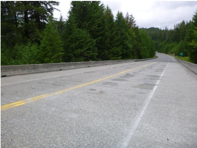
This bridge on US 12 over the Clear Fork of the Cowlitz River shows patching and potholing and needs resurfacing.
