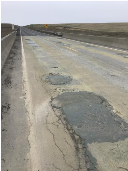
The Providence Coulee Bridge deck is deteriorated, with patching, cracking and spalling throughout. Replacing the top 3” of concrete will extend the bridge life. Left unaddressed exposes the entire deck to more deterioration, and the entire deck will need to be replaced.
