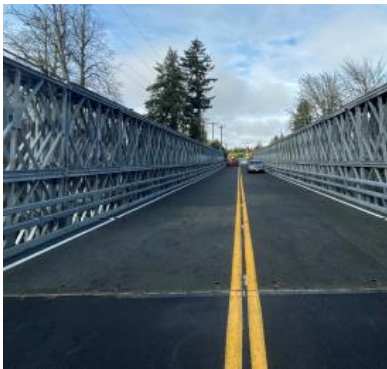
SR 162 Spiketon Creek Bridge: Bridge was closed in 2018, and an acrow temporary bridge was installed over the existing bridge in 2019 for $3.6 million. The old bridge still needs to be removed and replaced. This work does not prioritize at current funding levels, but may be required in conjunction with adjacent fish barrier corrections.
