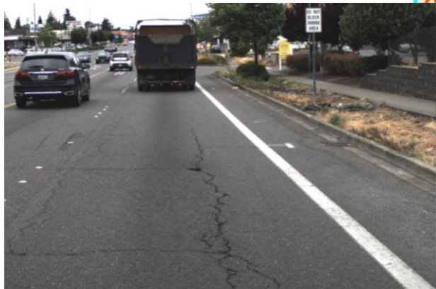
SR 7: Pavement cracking and potholes have reached a point where rehabilitation is needed now. There are also multiple expansion joints needing replacement at the north end of SR 7.
