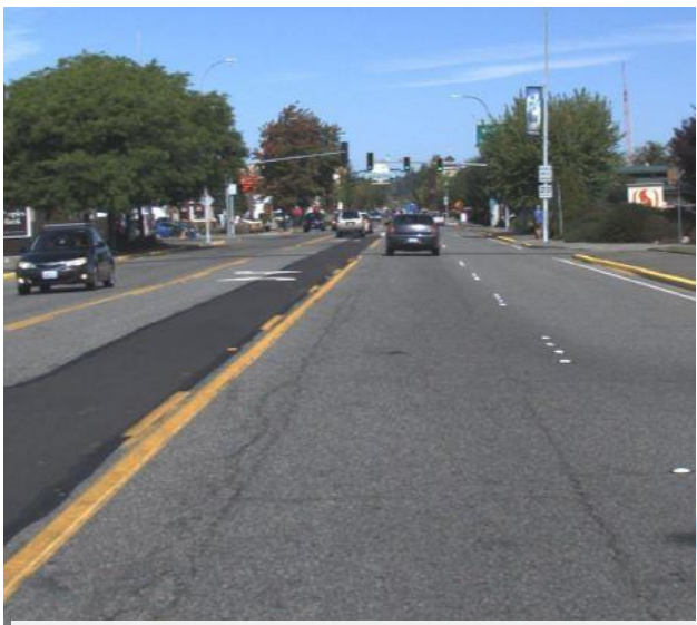
Last paved in 1997, extensive cracking and patching on State Route 20 Spur through Anacortes.
