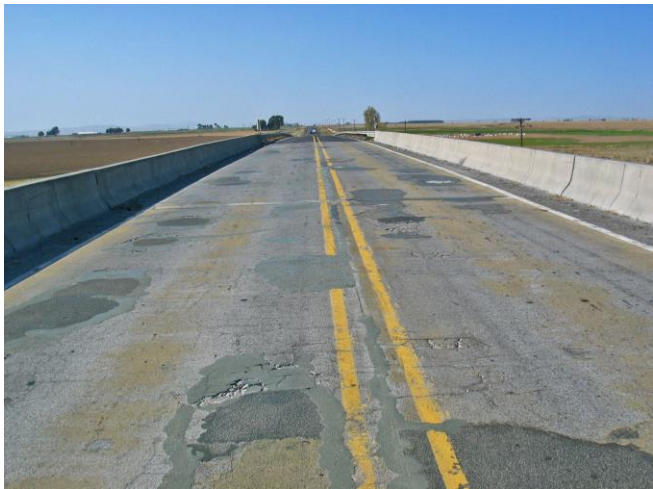
This bridge over the Koren Railroad is deteriorated with patching, cracking and spalling throughout.
