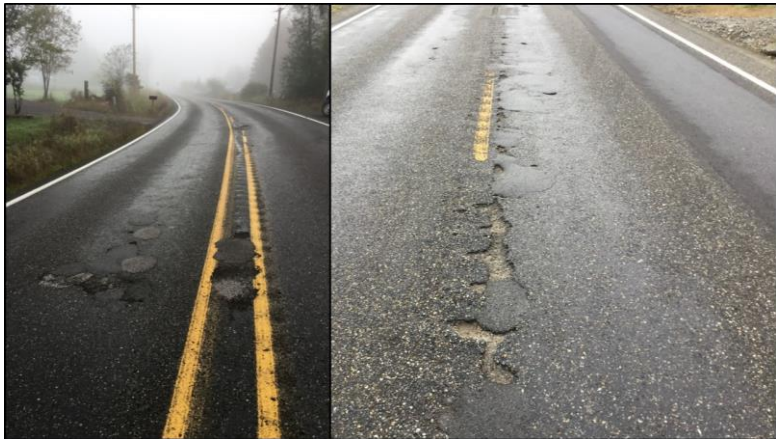
Cracking and delamination on State Route 508. In addition to the pavement structure being at risk, deteriorated pavements make it much more costly or even prohibitive to keep rumble strips in place. Major rehabilitation will be required if not addressed in ten years, and the need for full reconstruction is likely.
