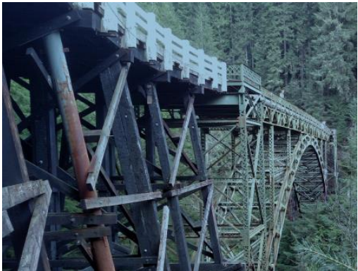
SR 165 Carbon River Bridge: Steel components need painting. Rust blooms throughout the rivets and plates, with some starting on stringers and floor beams. This sections also needs paving in the next ten years.
