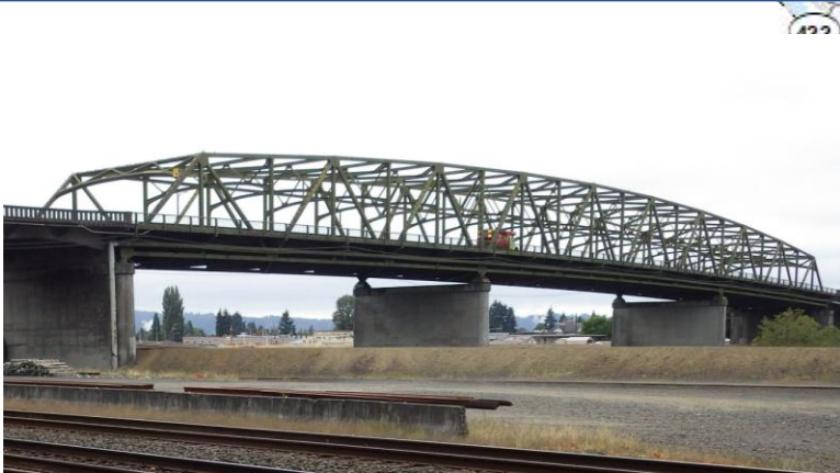
The Cowlitz River bridge on State Route 4 in Kelso is in need of painting and expansion joint repair.
