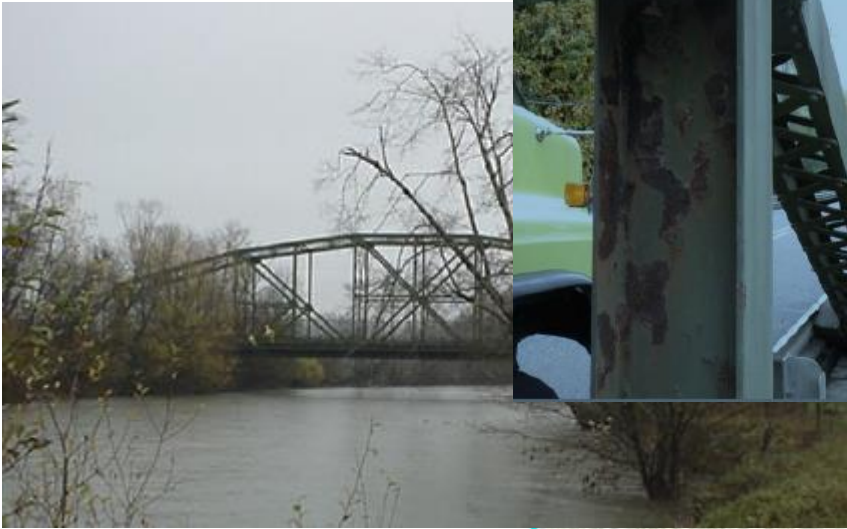
This bridge on US 101 over the Skokomish River has areas of chipped or peeled paint with some rust spots and staining. Steel members are starting to experience section loss.
