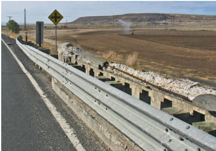
State Route 28 Crab Creek Bridge shows deteriorated concrete with exposed rebar and need to be replaced.
