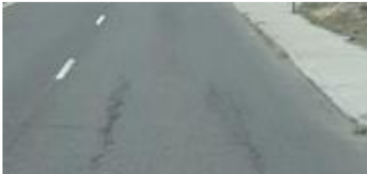
Pavement cracking in wheel paths on State Route 291.
