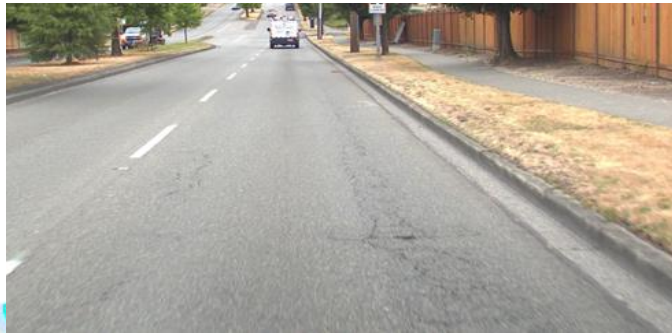
SR 163: Pavement cracking and potholes have reached a point where reconstruction is likely.
