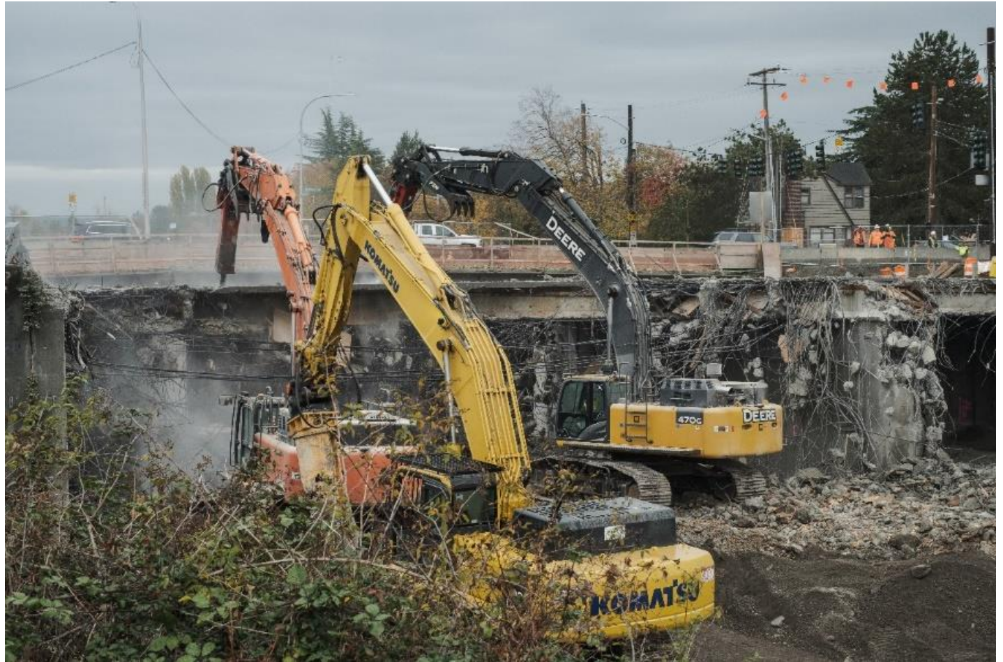
Removing Montlake Boulevard overpass – Oct. 23, 2021.
