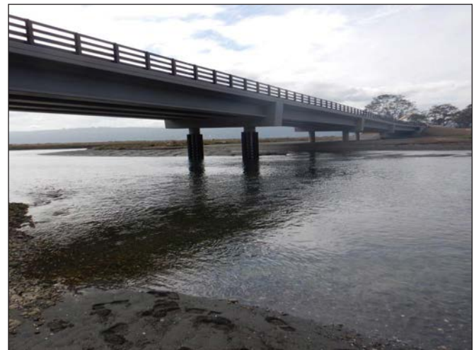
Figure 19. The new crossing is a multi-span bridge totaling approximately 410 ft (124.9 m). The reconstructed channel includes a tidal marsh area and a navigable connection for small craft between Oak Bay and Kilisut Harbor.
