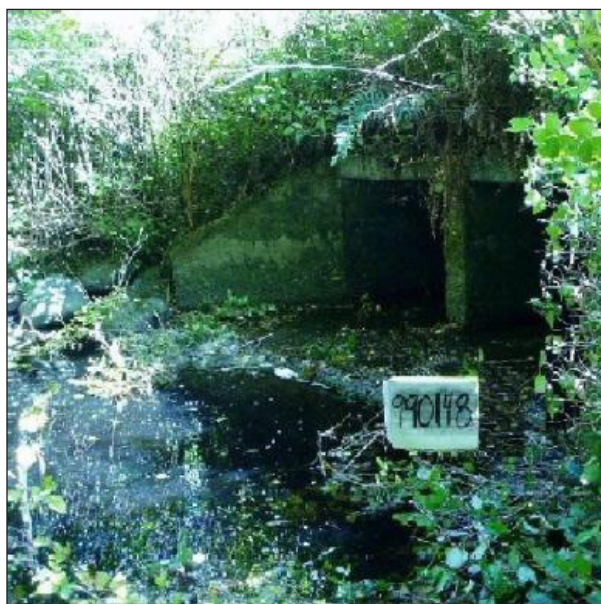
Figure 24. The old crossing was a double 5 ft (1.52 m) by 4 ft (1.22 m) concrete split box culvert that was a barrier due to high velocity and low water depth at fish passage flows.
