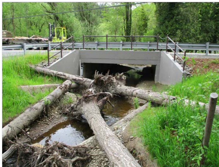
Figure 11. The new culvert is a 16.1 ft (4.9 m) wide by 9 ft (2.74 m) high concrete box culvert. Abundant large wood was placed both upstream and downstream of the new culvert to provide deep resting pools and refugia for fish.
