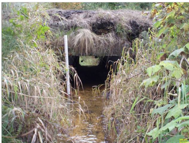
Figure 10. The old culvert was a 5 ft (1.53 m) wide by 3 ft (0.91 m) high concrete box culvert that was a high flow velocity barrier to migrating chum, coho, steelhead, and sea-run cutthroat trout.
