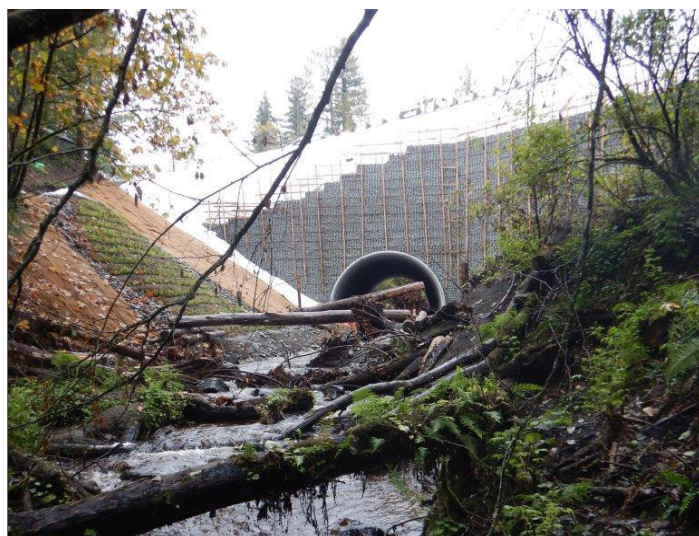
Figure 9. The new structure is a 26 ft (7.9 m) diameter structural plate steel culvert fitted with boulder cross-vanes to force the formation of step pools. Outside the structure, large wood and small slash were incorporated into the stream channel design. A deformable grade control, created with woody branches, helps to dissipate stream energy and reduces velocity entering the project reach.
