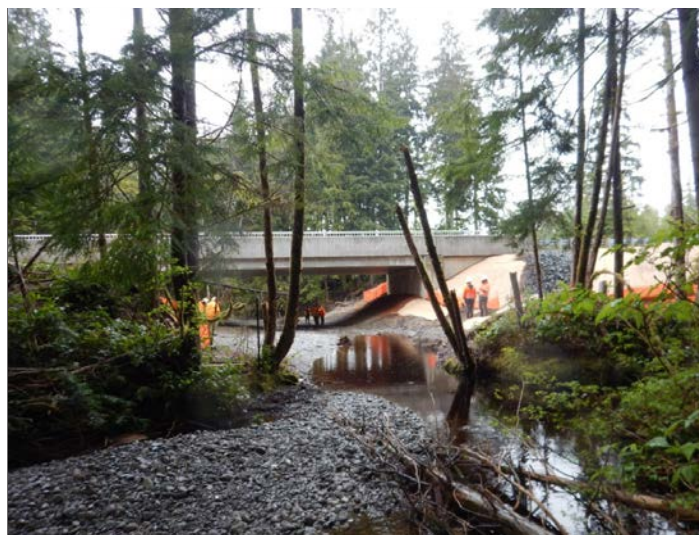
Figure 25. The new crossing on US 101 is a 63 ft (19.24 m) span concrete bridge that restores access to 3.19 mi (5.13 km) of habitat for chum, coho, steelhead, sea-run cutthroat, and bull trout.
