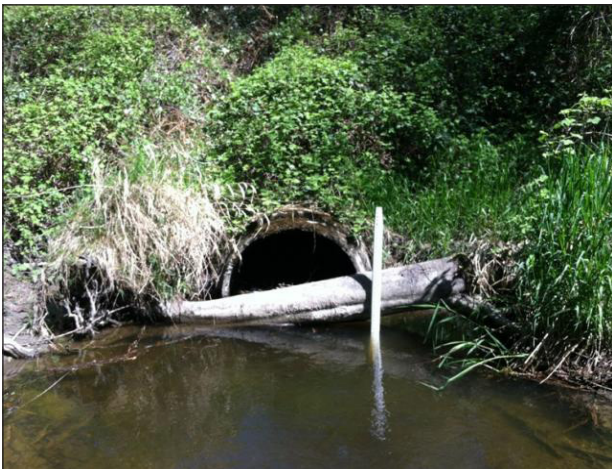
Figure 14. The old crossing for Loutsis Creek was a 4 ft (1.22 m) diameter concrete culvert that was a slope barrier.
