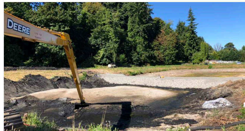
Figure 6. A stormwater pond in WSDOT's southwest region is cleaned to keep the pond functioning as designed.
