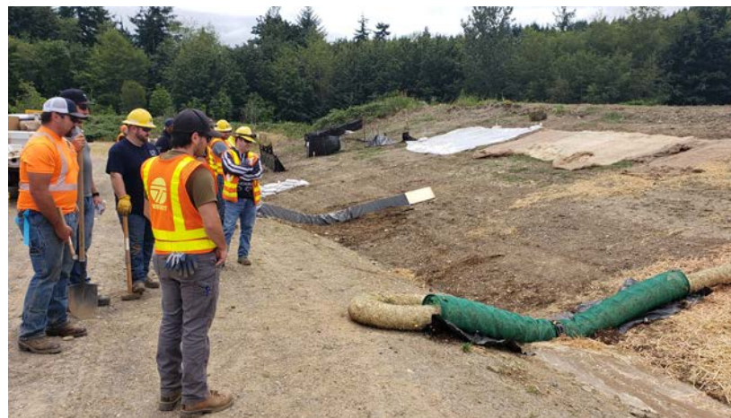
Figure 4. Participants from WSDOT's field BMP training test check dam effectiveness.
