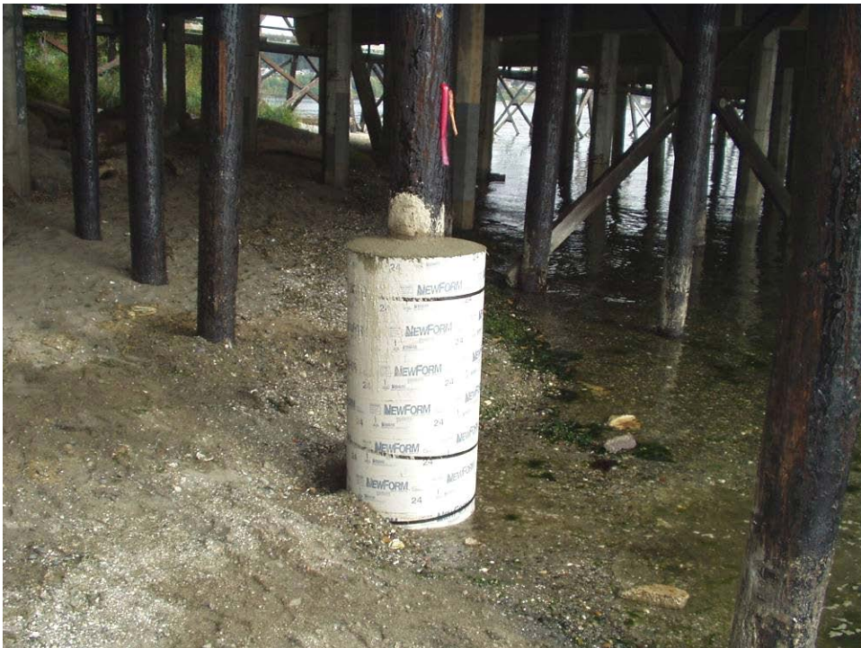
Figure 2-19 Completed Pile Encapsulation
