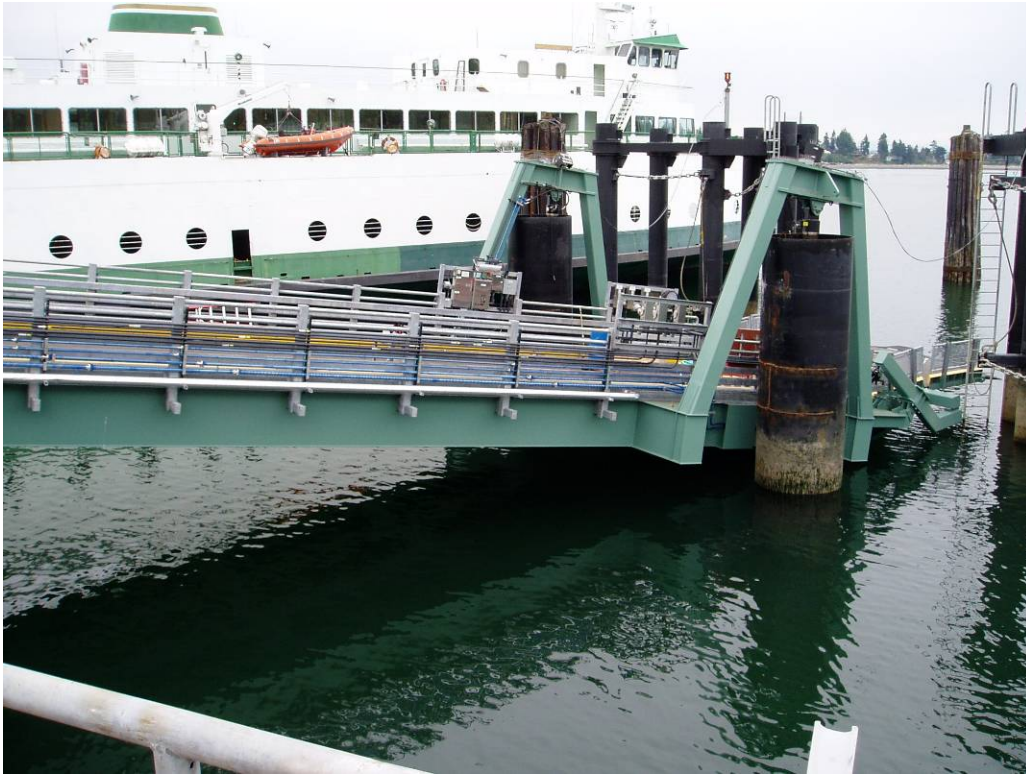
Figure 2-38 Compression Cylinder Tower System
