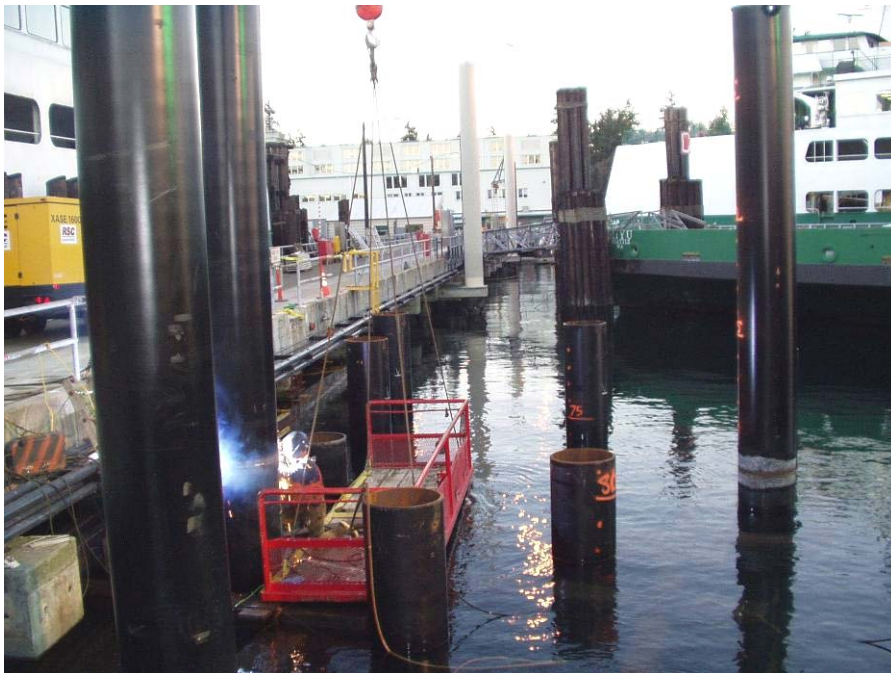
Figure 2-21 Bent Steel Pile in Need of Repair
