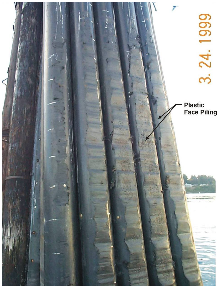
Figure 2-27 Plastic Face Piling on a Fixed Timber Dolphin
