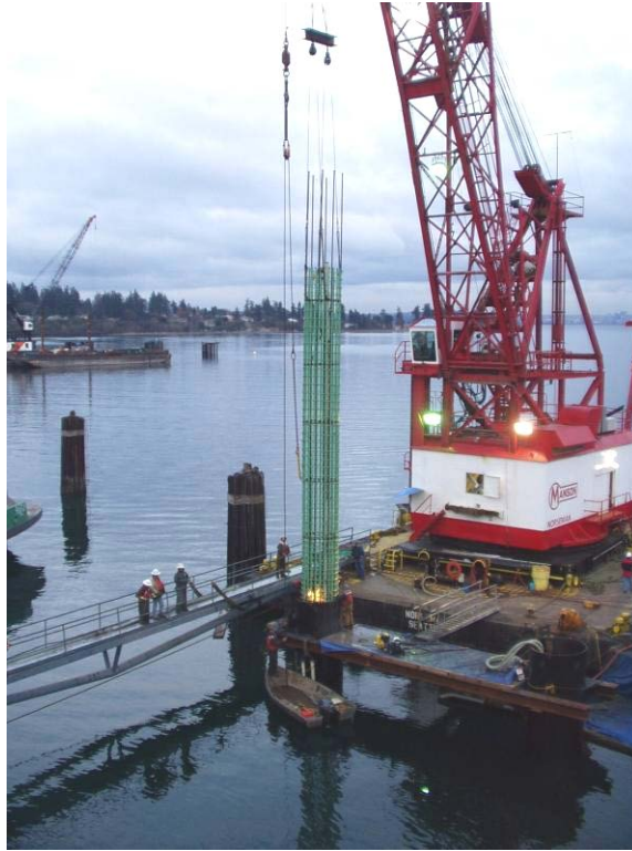
Figure 2-11 Rebar Reinforcement of Drilled Shaft
