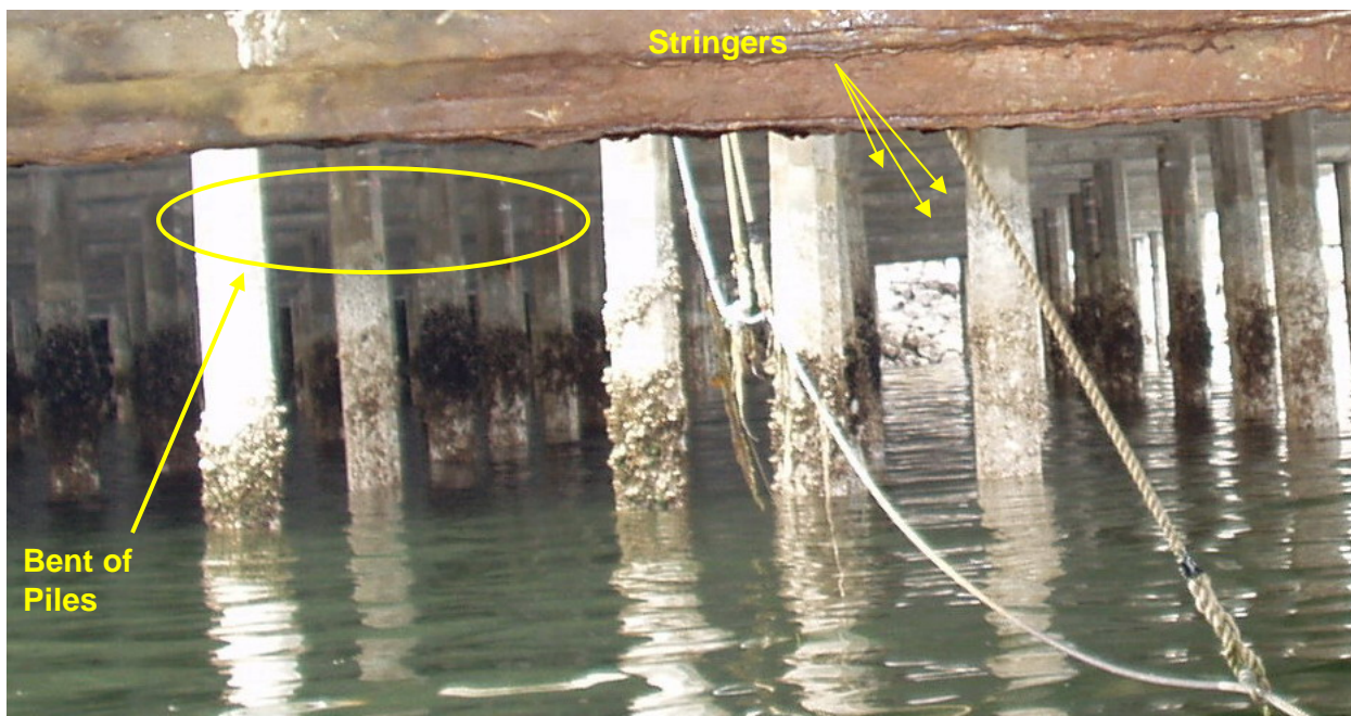
Figure 2-42 Under a Timber and Concrete Trestle
