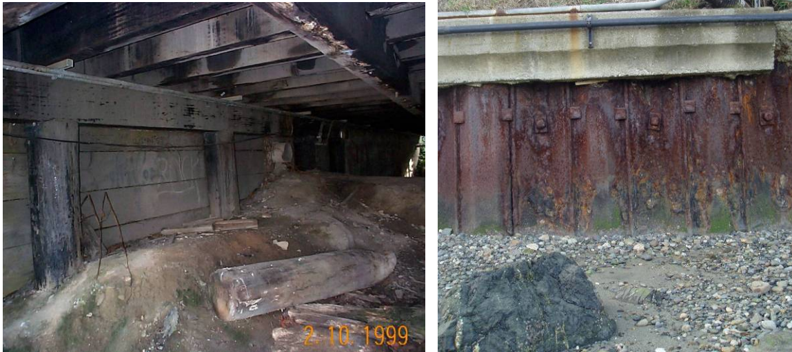
Figure 2-49 Timber and Steel Bulkheads
