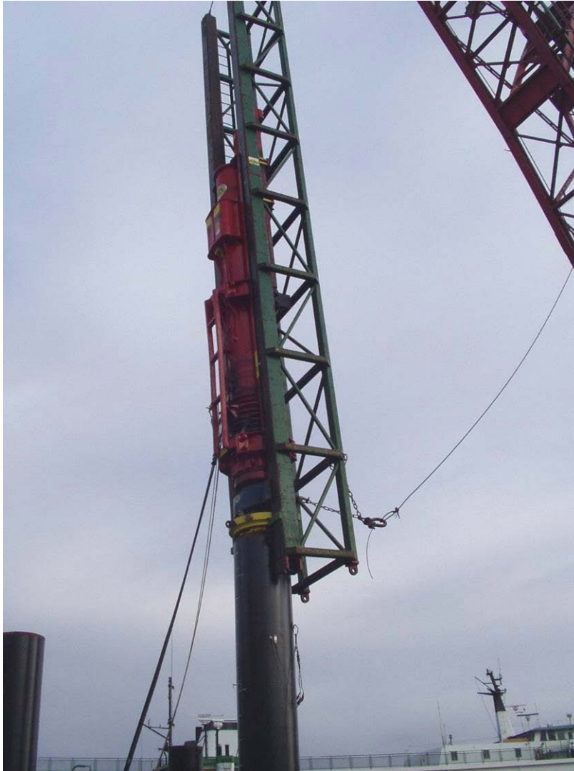
Figure 2-4 Impact Hammer Driving a Steel Pile
