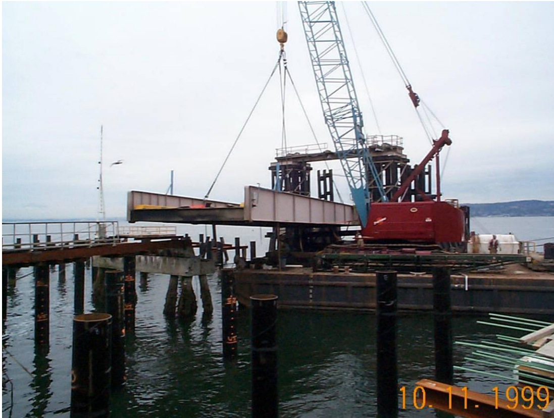
Figure 2-39 Removal of a Transfer Span
