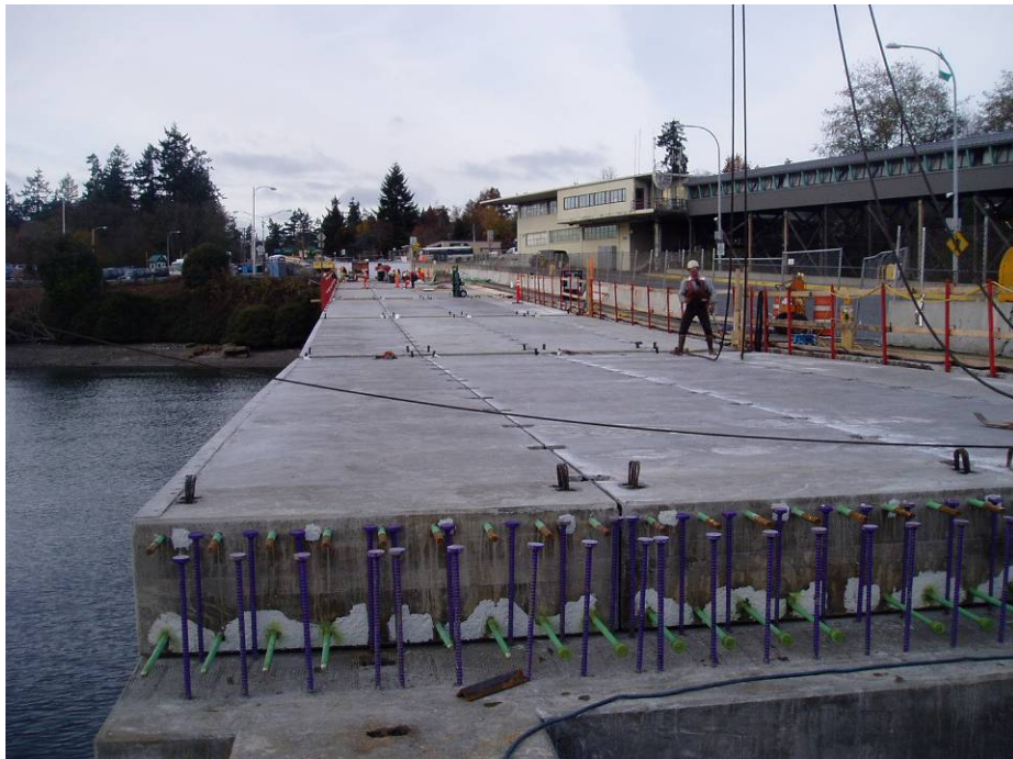
Figure 2-46 Pre-cast Concrete Deck Panels
