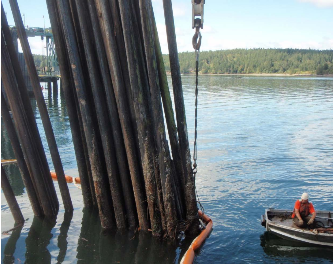
Figure 2-2 Direct Pull of Timber Piles
