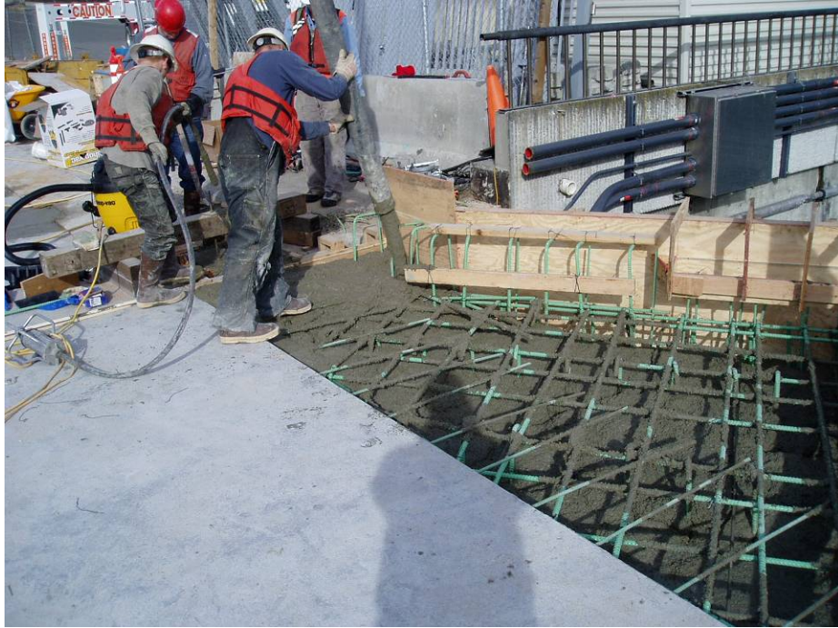
Figure 2-45 Pouring Concrete for Cast-in-place Deck Panels
