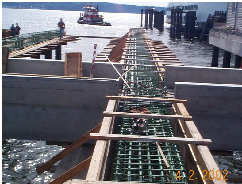
Figure 2-41 Forms Used for a Cast-in-place Concrete Pile Cap
