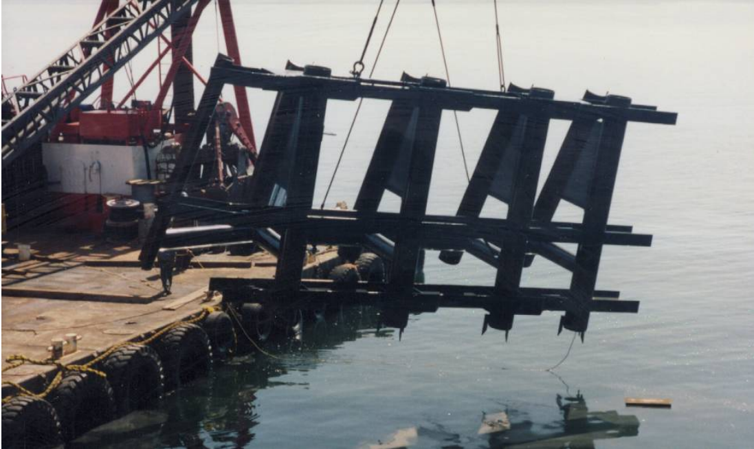
Figure 2-37 Crane Installing Steel Wingwall Frame
