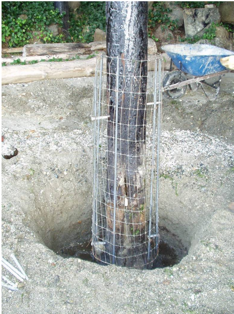
Figure 2-17 Pile Prepared for Encapsulation
