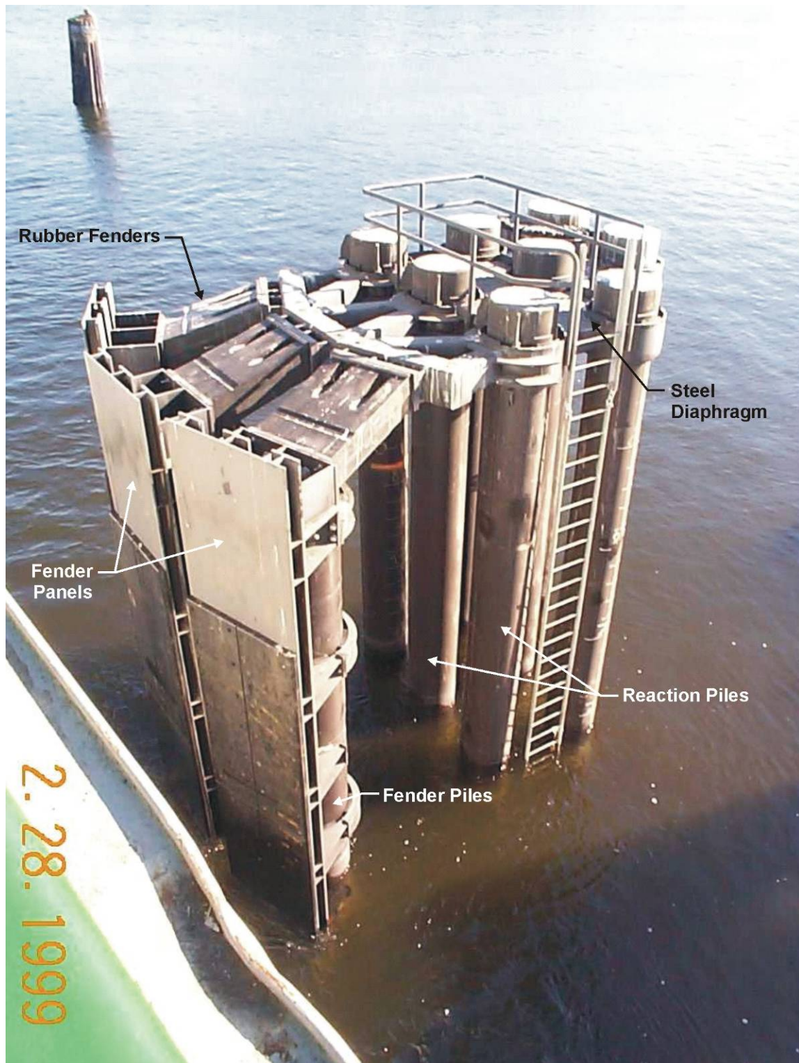
Figure 2-31 Typical Steel Dolphin
