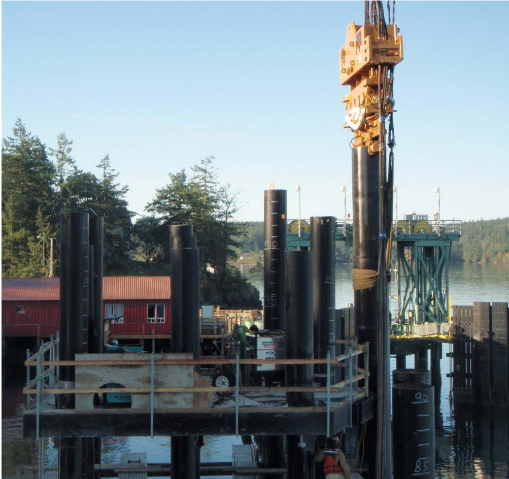
Figure 2-5 Vibratory Hammer Installing a Steel Pile
