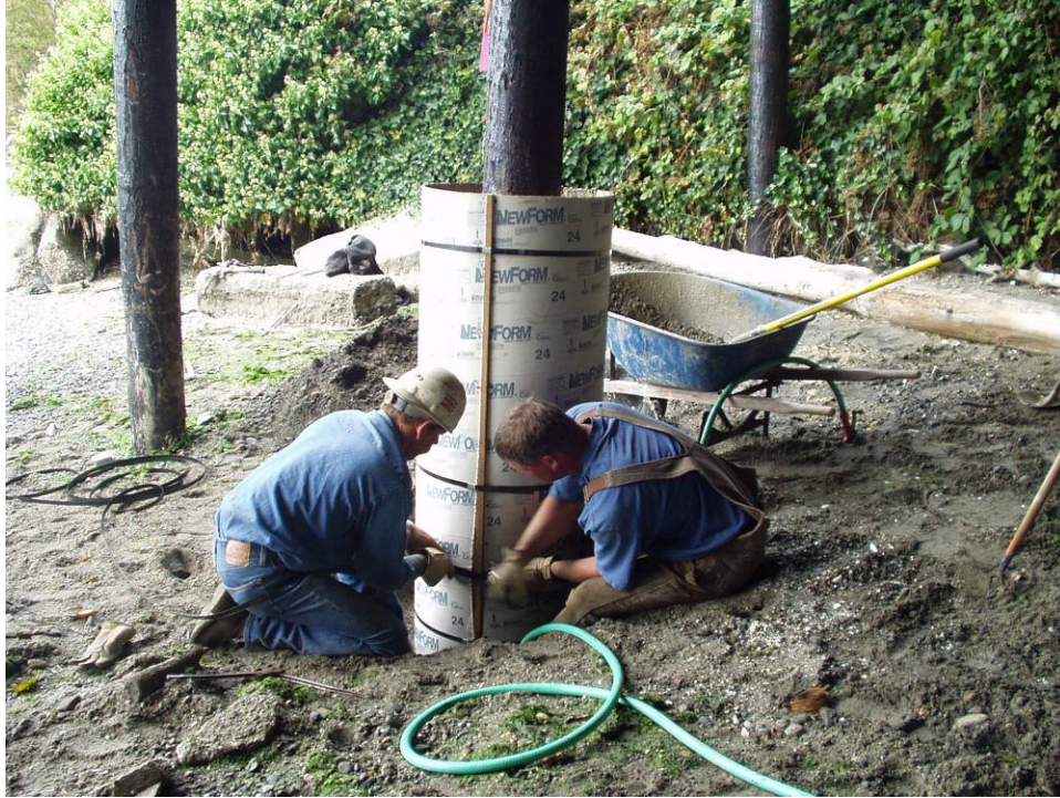
Figure 2-18 Installing the Form
