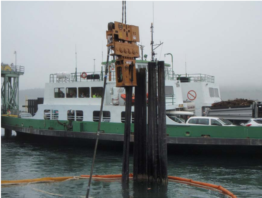
Figure 2-1 Vibratory Hammer Removing a Timber Pile
