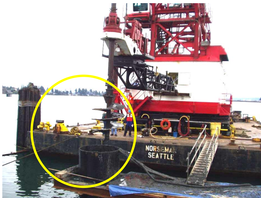
Figure 2-10 Auger Excavation of Drilled Shaft
