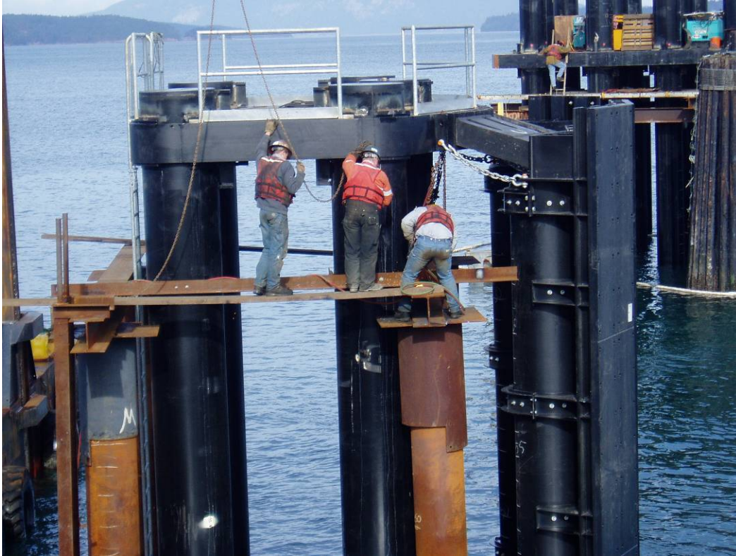
Figure 2-51 Work Platform Supported by Temporary Steel Piles
