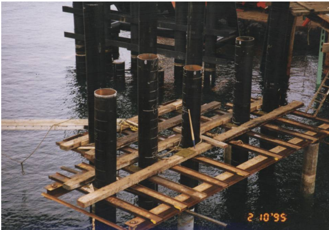
Figure 2-36 Template Used During Steel Wingwall Installation
