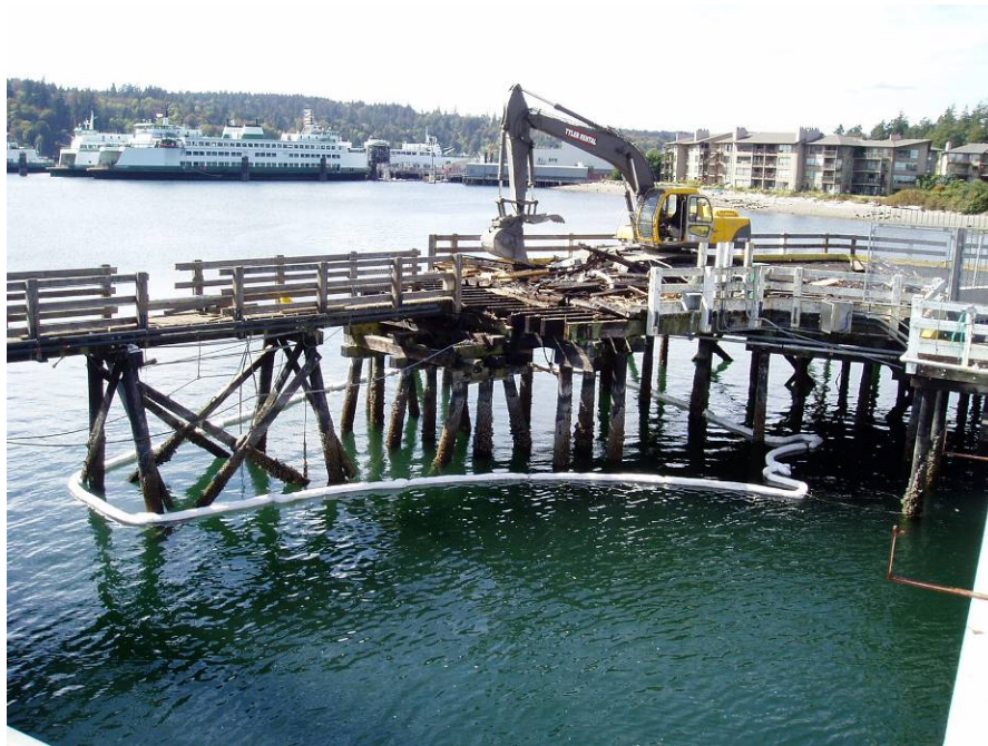
Figure 2-43 Removal of Timber Decking
