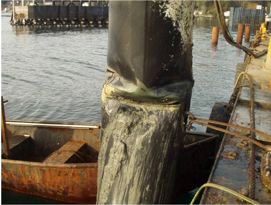
Figure 2-21 Bent Steel Pile in Need of Repair
