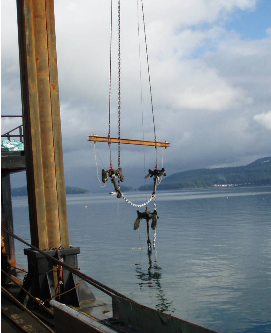
Figure 2-29 Installation of Floating Dolphin Anchors
