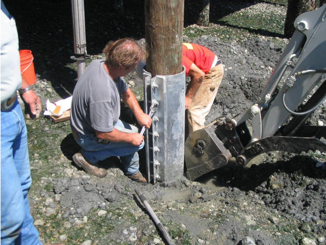
Figure 2-15 Pile Stubbing: Steel Collar Method
