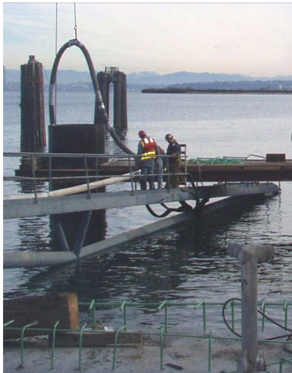
Figure 2-12 Vacuuming of Slurry from Drilled Shaft
