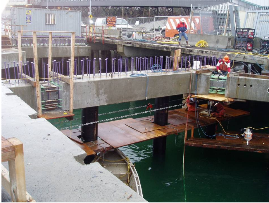
Figure 2-44 Concrete Pile Cap
