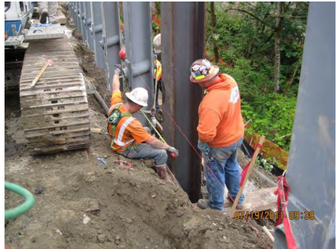
Figure 4. Retaining wall being installed on SR 9 to avoid wetland impacts
