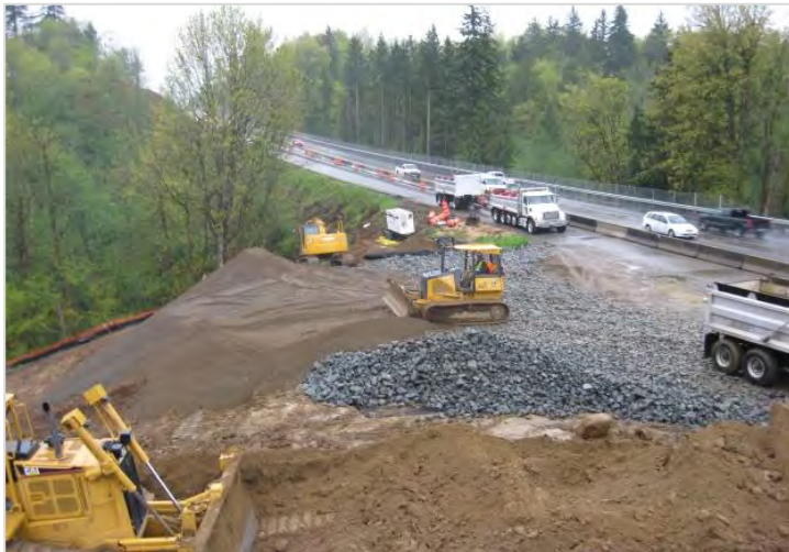
Figure 16. Construction of pad for stormwater vault
