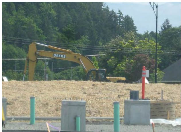
Figure 1. Straw used as a temporary mulch to prevent erosion
