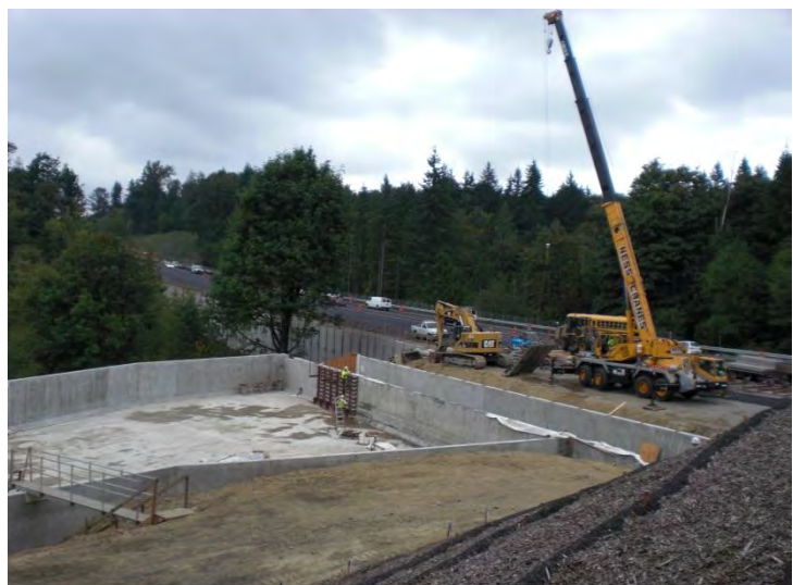
Figure 17. Stormwater vault
