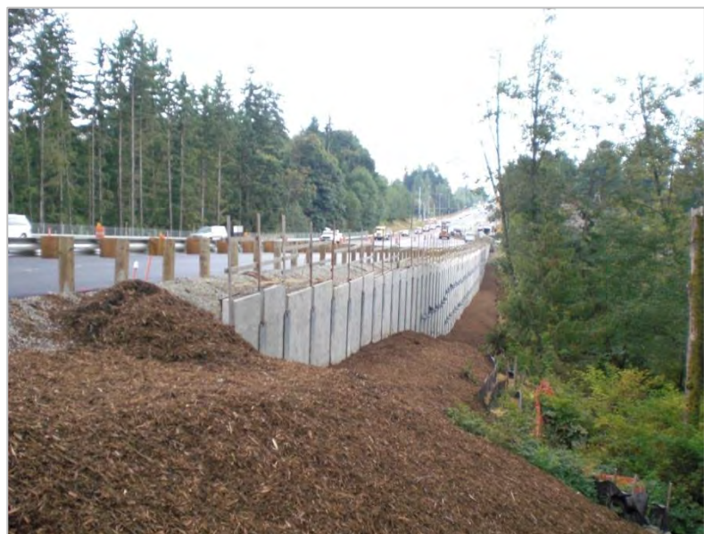
Figure 15. Retaining wall installed to avoid wetland impacts
