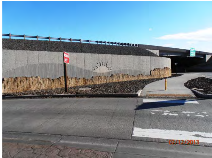
Figure 10. Context Sensitive Solution treatment on retaining wall on I-82 – Valley Mall interchange
