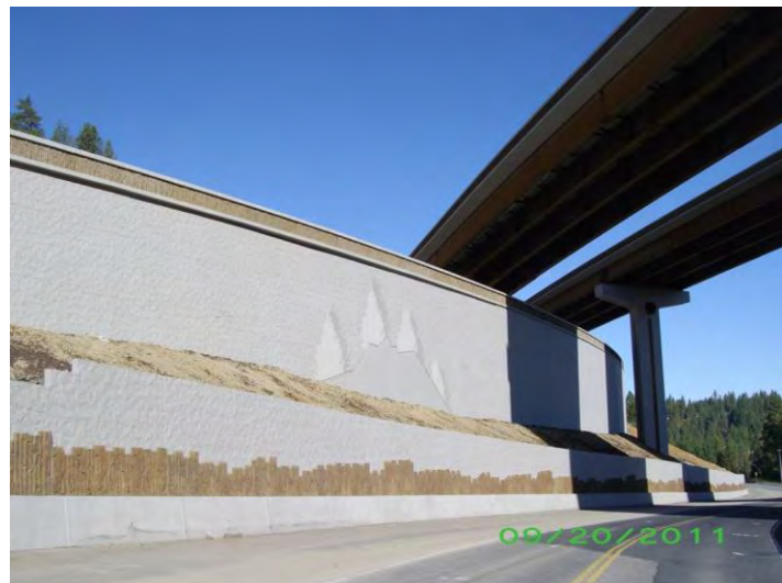
Figure 11. Context Sensitive Solution treatment on retaining wall and bridge columns on SR 395/US 2
