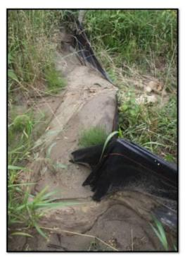
This silt fence breach illustrates the need for proactive source control and Temporary Erosion and Sediment Control (TESC) planning on construction projects.
