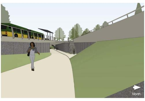
View of passageway below Montlake Boulevard East with clear views of the exit beyond, tunnel users and activity at street level. The access stair landing is set back from the path of travel to provide adequate space for users to comfortably enter and leave the pathway.
