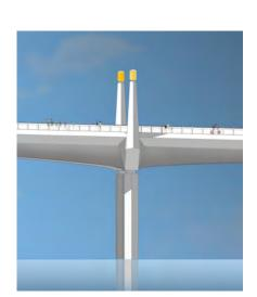
**Box girder:** Portage Bay Bridge elevation of box girder bridge with shared-use path looking north from Montlake Playfield.
