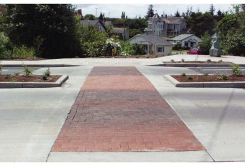
A raised crosswalk with specialty paving to alert motorists to crossing in Port Townsend, WA. (Source: SvR Design Company)
