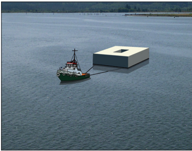
Step 2: Tow pontoons from construction facilities to the Lake Washington area.
