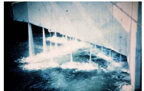
Fluke anchor with water jets to help embed the anchor into lake bottom.
