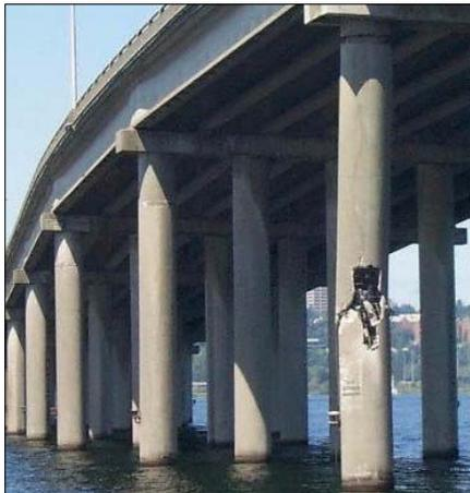
**Exhibit 2.** Hollow columns support the floating bridge approaches, shown here damaged by a barge in 1999.
