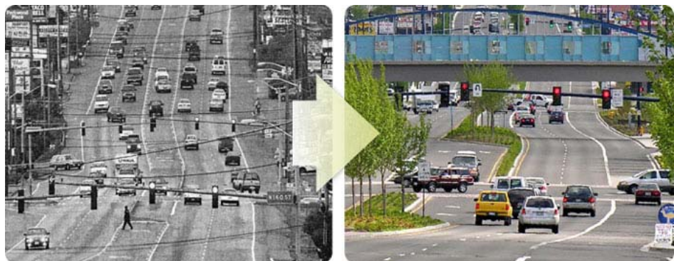
These before and after photos from the Aurora Avenue Project (Shoreline, Washington) illustrate how successful CSS projects improve safety and mobility for a variety of users. The photo illustrates a new grade-separated pedestrian crossing, improved sidewalks, managed access, enhanced greenscape.
