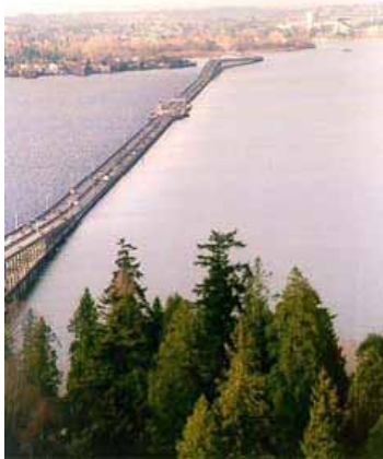
View of aerial view of bridge, looking west from Medina taken
