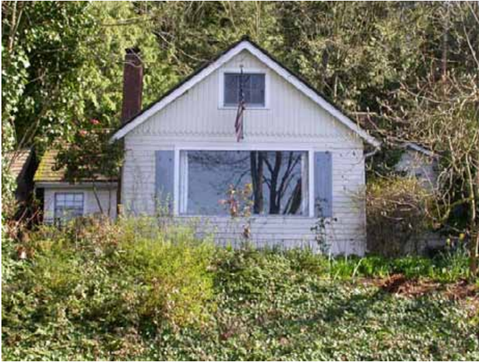
View of west elevation that faces Lake Washington taken 3/8/2004
