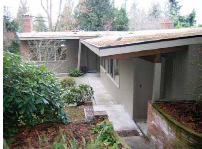
View of east and south elevations taken 1/22/2009
