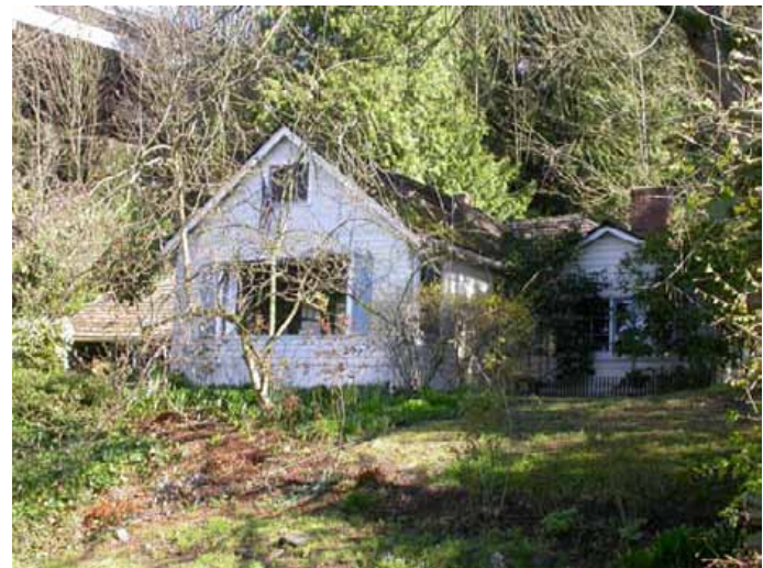
View of West and south elevations taken 3/8/2004
