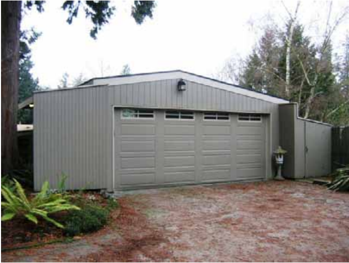
View of east elevation of garage, facing Evergreen Point Road taken 1/22/2009
