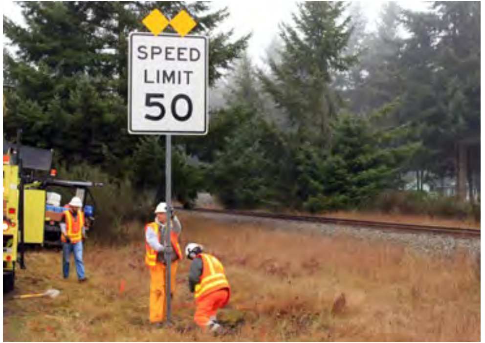
WSDOT crews installed reduced speed limit signs along a three mile section of US 12 near Rochester.
