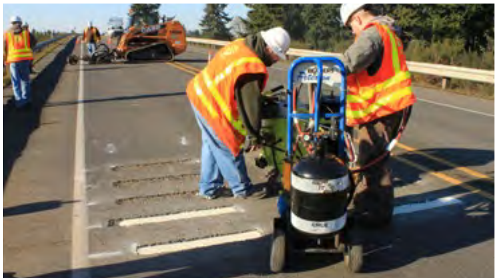
Back filling rumble strips with plastic west of Pecan Street SW.
