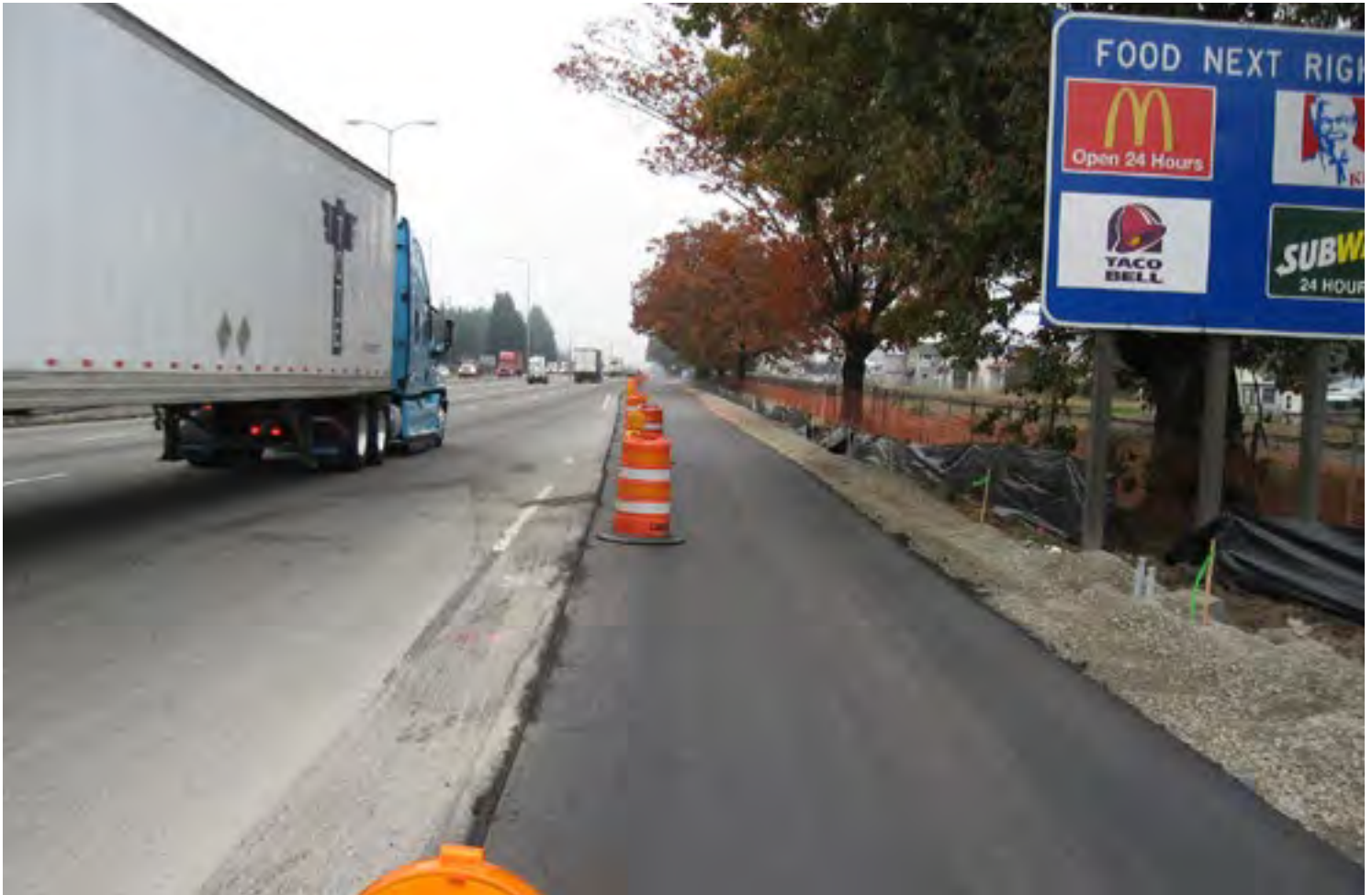
I-5 auxiliary lane under construction.
