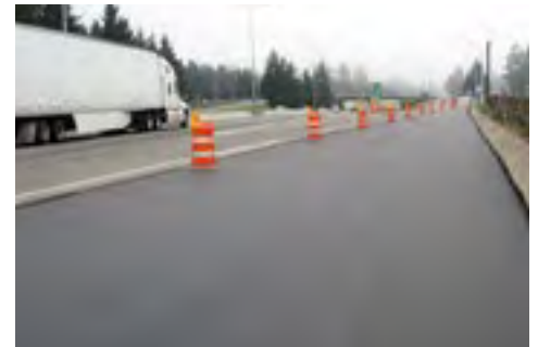
I-5 auxiliary lane under construction.
