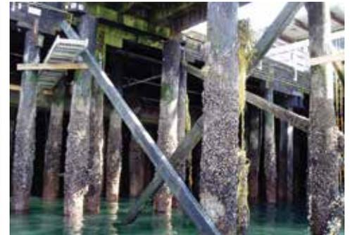
*Clockwise from left: Aerial view of construction at Colman Dock, June 2019; an example of a deteriorating timber pile that has been removed and replaced at Colman Dock; existing timber trestle will be replaced with new concrete and steel trestle.*
