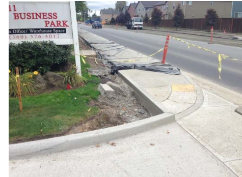
Clark County: NE 10 th Av. Construction
