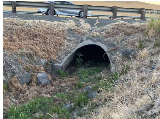
Figure 2. A Culvert at US 195 Washington State
