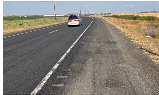
Figure 7. Highway Shoulder at US 12
