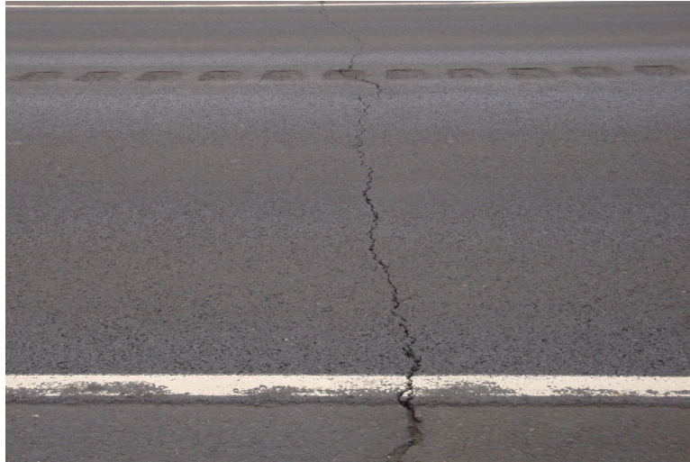
Exhibit 3-2 Transverse Cracking
