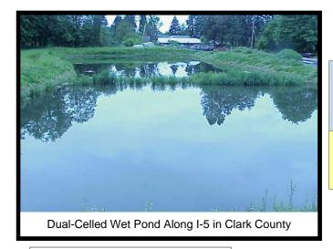
**Description:** Stormwater pond that retains a permanent pool of water (wet pool), at least during the wet season.
