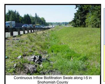
**Description:** Variation of basic biofiltration swale. Water enters swale continuously along side slope. The basic Biofiltration design is modified by increasing swale length to achieve an equivalent average hydraulic time.
