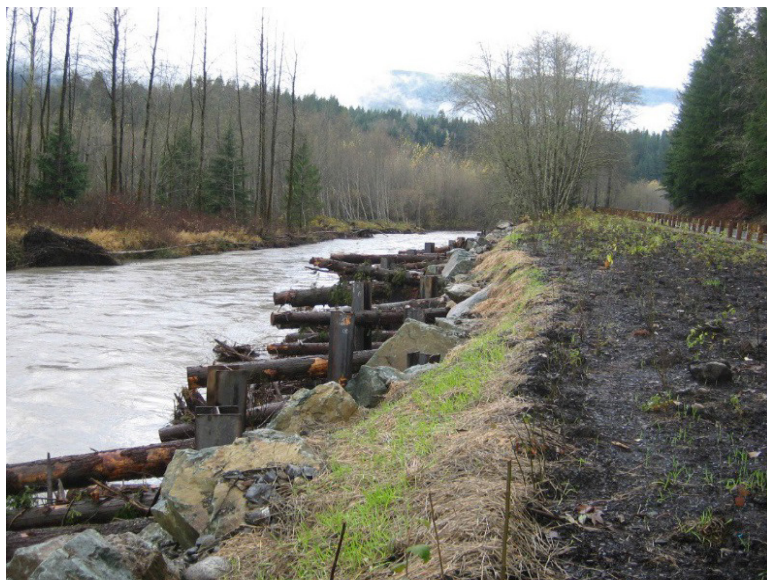
Figure 10A-6 Crib Wall with Soil Lifts (No Piles), Sauk River, Snohomish County
