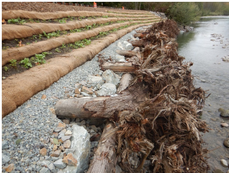
Figure 10A-6 Crib Wall with Soil Lifts (No Piles), Sauk River, Snohomish County
