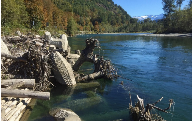
Figure 10A-9 Dolotimber Structures, Skagit River, Skagit County
