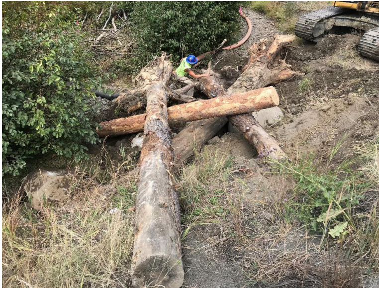
Figure 10A-1 Self-ballasting Large Wood Structure, Swauk Creek, Kittitas County
