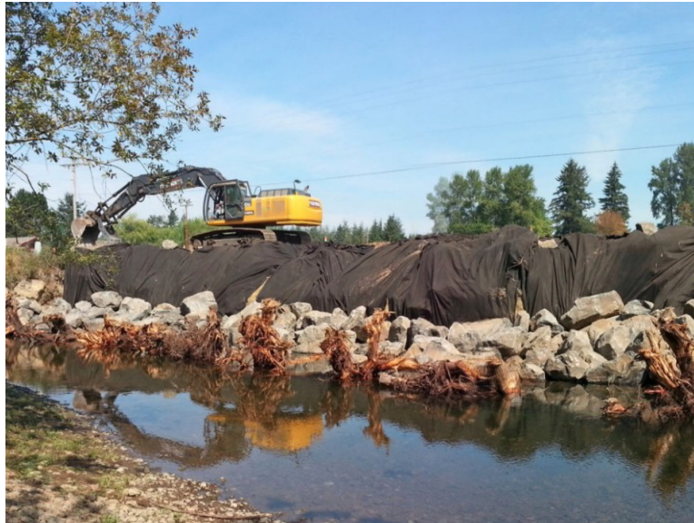
Figure 10A-3 Wood-Studded Revetments, Newaukum River, Lewis County
