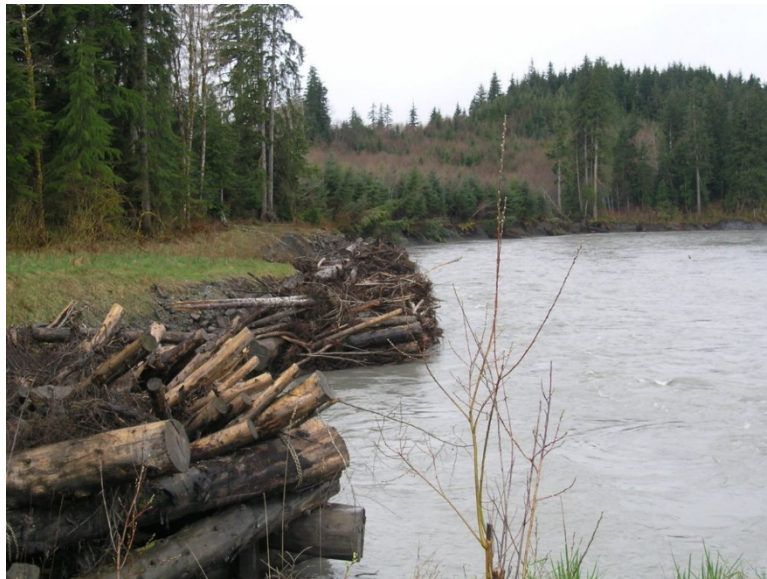
Figure 10A-7 Flow Deflection Jams, Hoh River, 2004, Clallam County
