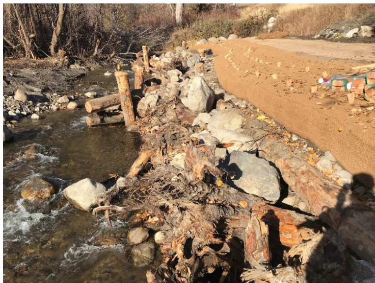
Figure 10A-4 Crib Wall with Wood Piles, Beaver Creek, Okanogan County
