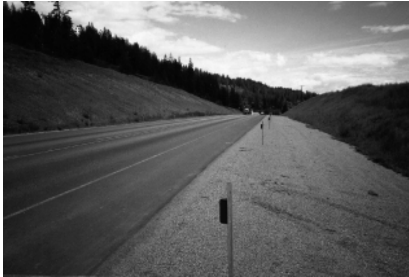
Wildlife Reflectors on a Tangent Section Figure 830-3
