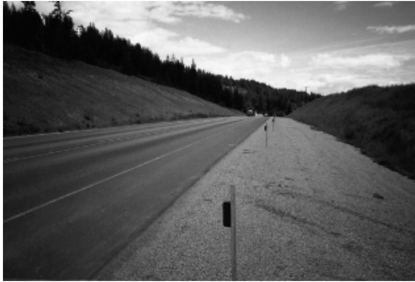
Wildlife Reflectors on a Tangent Section Figure 830-3
