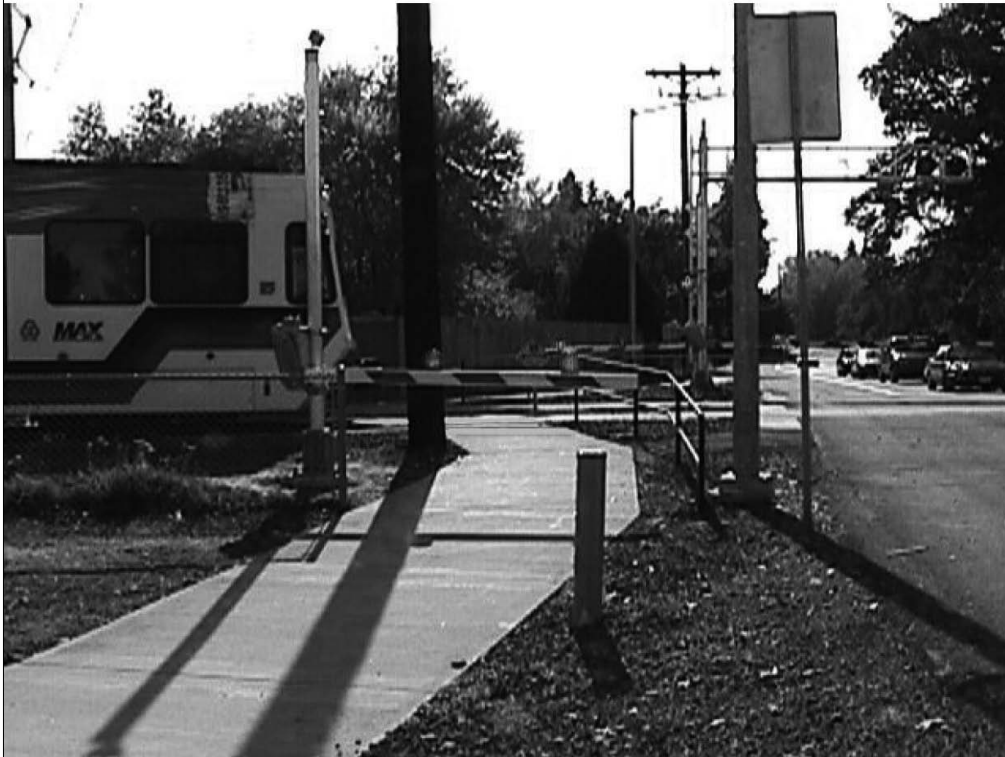
Pedestrian Railroad Warning Device Exhibit 1510-17
