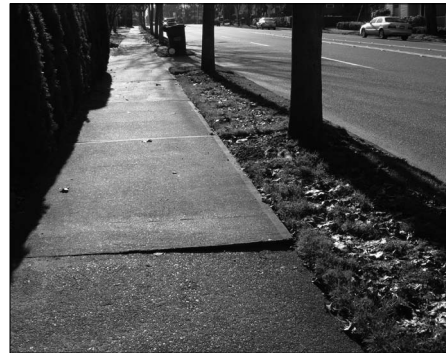
Unacceptable Pedestrian Access Route
