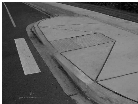
Perpendicular Ramps
