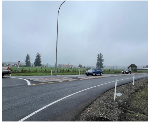
Splitter Island cut through on State Route 530 at 59 th Ave NE
