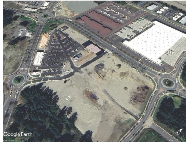
Access Management - Marvin Rd NE and Willamette Dr, Lacey WA (Source: Google Earth)
