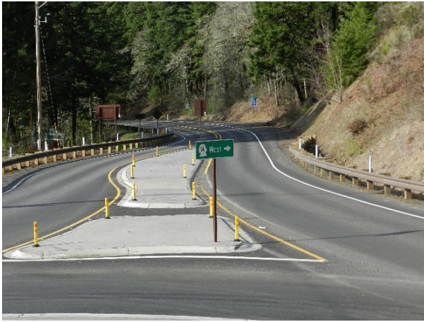
Splitter Island cut-through on State Route 14 at Wind River Highway
