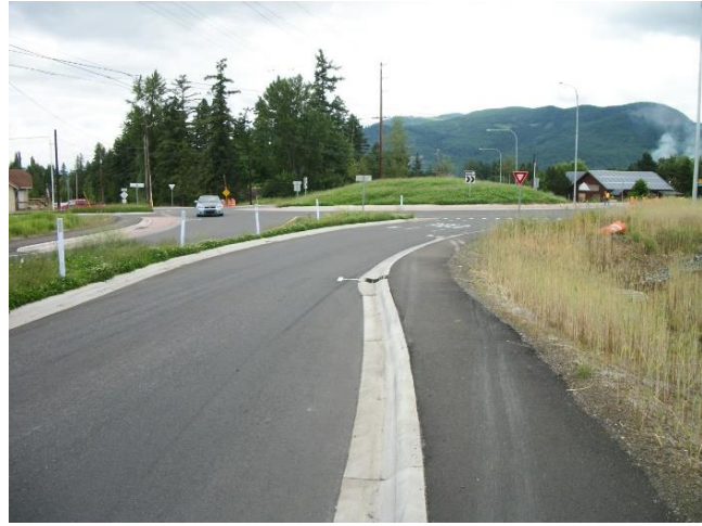
Rolled curbing on SR542 at East Smith Rd
