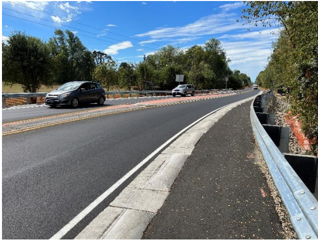
Raised curbing with gaps for drainage on State Route 500 at 182 nd Ave.
