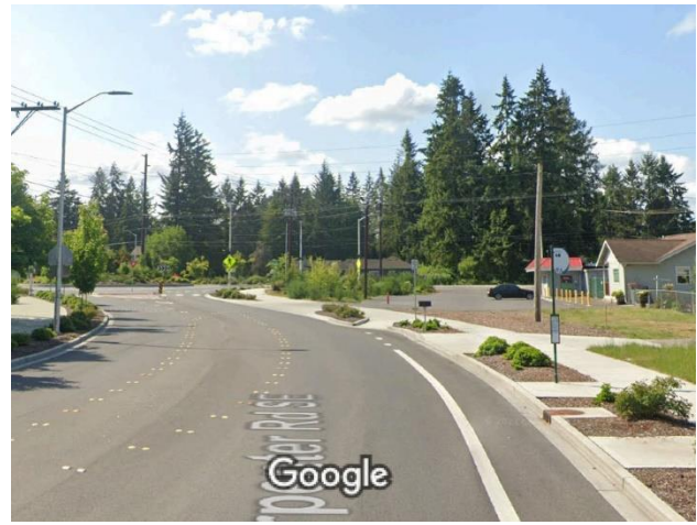
In-lane transit stop on near side of roundabout approach – Carpenter Rd SE, Lacey WA (Source: Google)
