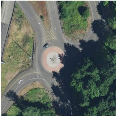
Roundabout showing two-color mountable central island. Location is State Route 432 at Exit 36 on Interstate 5 in Kelso, WA
