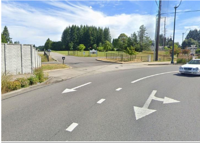
Driveway approach within circulating area - Yelm Hwy SE, Olympia WA (Source: Google)
