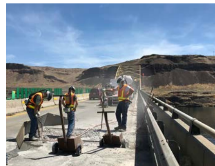
WSDOT bridge maintenance crews repair the deck of the I-90 Vantage Bridge over the Columbia River between Kittitas and Grant counties while adhering to COVID-19 safety measures.
