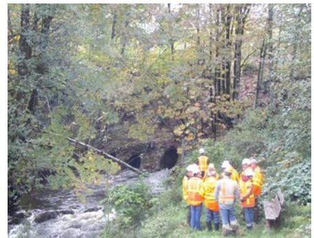
Before: The three culverts on Coffee Creek under US 101 were a barrier to fish passage. Scoping meeting at the Coffee Creek US 101 culvert outlet on October 3, 2013.
