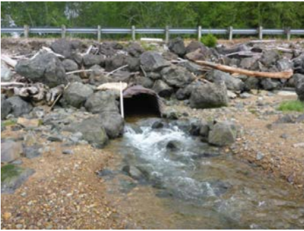
Before: The SR 401 old crossing at Hungry Harbor was a corrugated metal culvert 5 feet in diameter that blocked Chinook, coho, steelhead and sea run cutthroat from reaching upstream spawning habitat.
