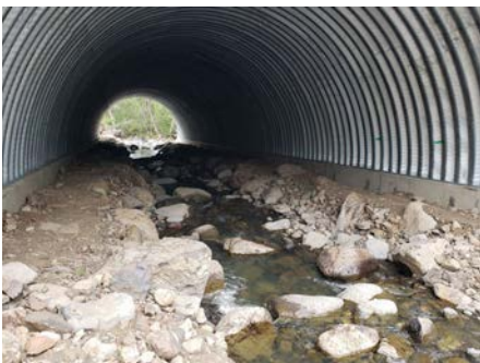
After: The culvert on Buford Creek at SR 129 was corrected to allow access to upstream potential spawning habitat for fish.
