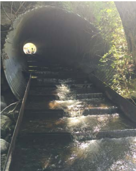
Before: The culvert on Buford Creek at SR 129 was a barrier to fish passage.
