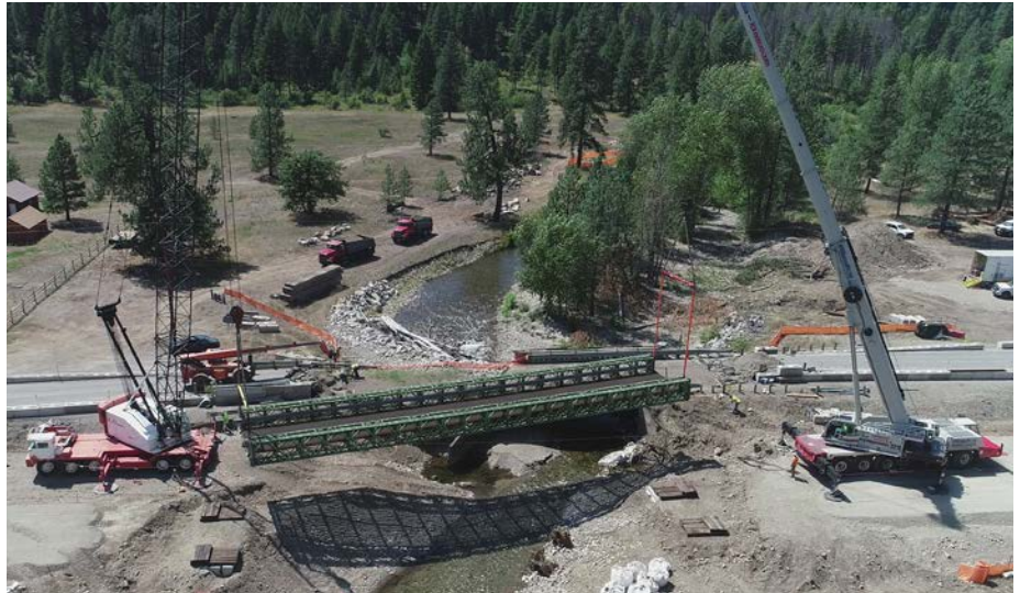
A Bailey bridge being moved to a temporary location at the Sanpoil River in 2019, which allowed WSDOT to build a new bridge at the location.
