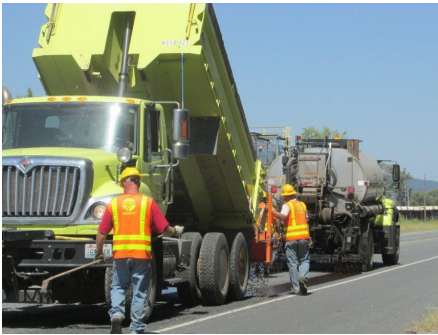
A WSDOT maintenance crew applies chip seal on U.S. Route 395. Chip seal, or bituminous surface treatment, is a cost-effective method used to extend the life of roads.
