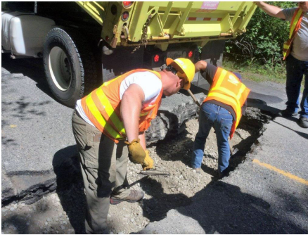
A WSDOT maintenance crew performs emergency repairs on State Route 534 after a sinkhole damaged the highway.
