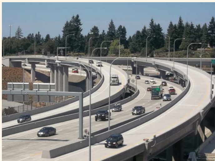
Drivers head toward Interstate 5 on new eastbound ramps and bridges constructed on State Route 16 in Tacoma's Nalley Valley.
