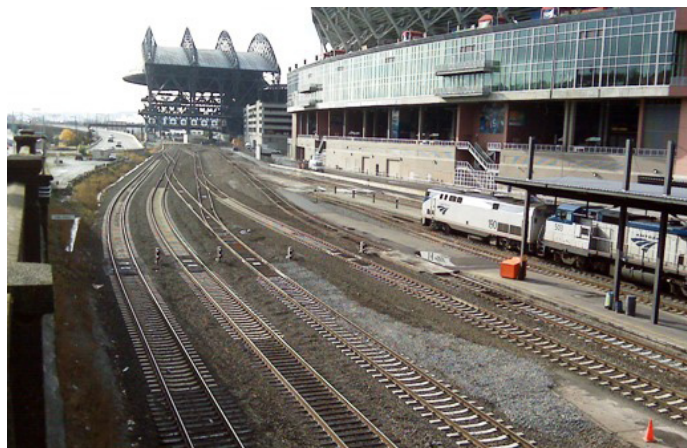
Fourth Avenue looking south shows the existing two mainline tracks, and connecting tracks at King Street Station.
