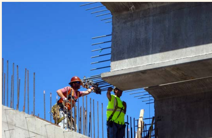
Crews work to move a large concrete girder into position on the Salmon Creek project in Clark County.
