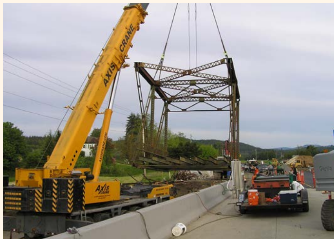
Crews use a crane to remove the superstructure of the old SR 6 Willapa River Bridge.
