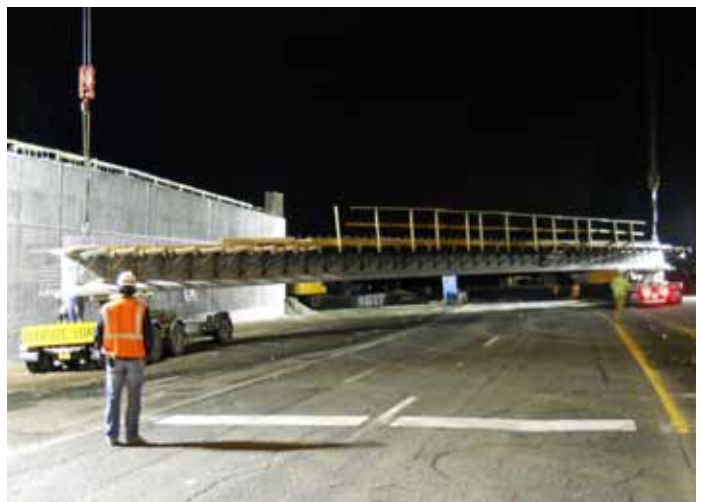
Crews closed the highway overnight while they installed seven 120-foot long girders into place over SR 500.
