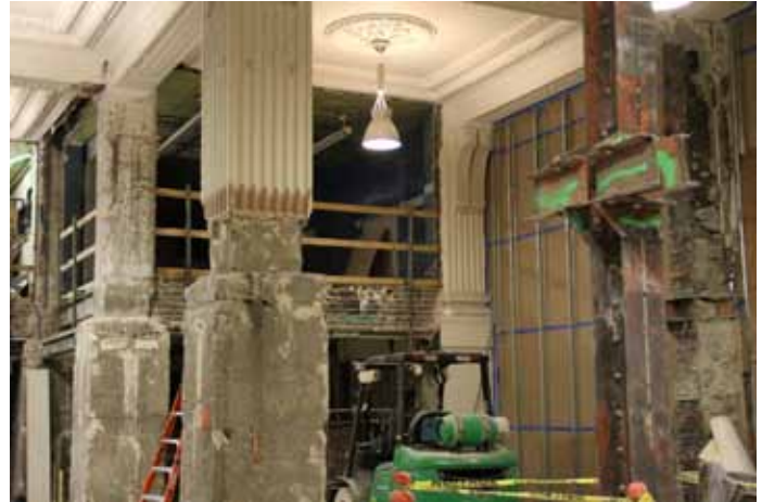
The exposed steel column (on the right) in King Street Station's main waiting area was stripped and prepared for added steel reinforcement to help the 100-year-old building better withstand earthquakes.
