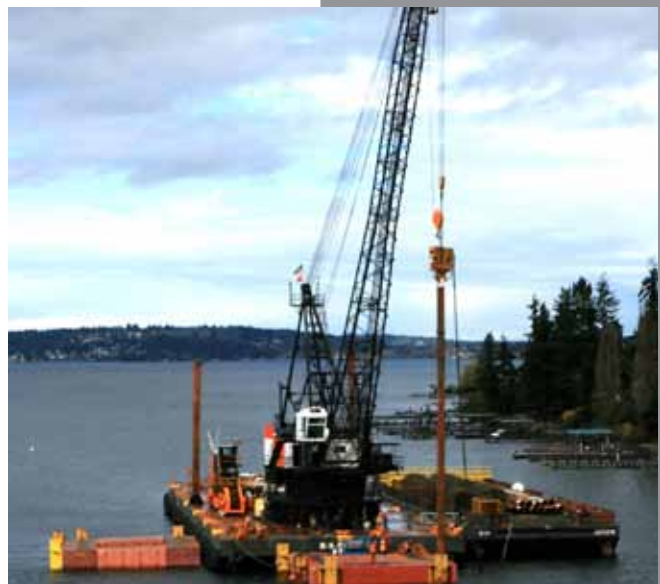
The barge and crane pictured here is preparing to install shaft anchors in Lake Washington for the new SR 520 floating bridge.
