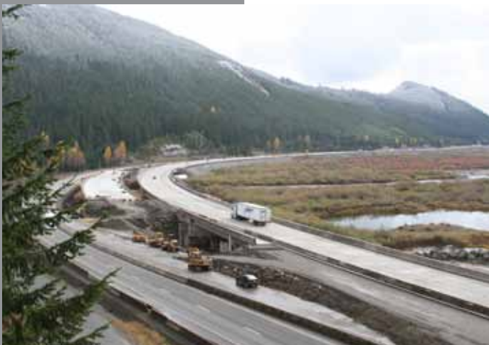
WSDOT opened the new eastbound lanes at Gold Creek during fall 2011. Crews are building the new westbound lanes this summer, which will open to traffic in the fall.
