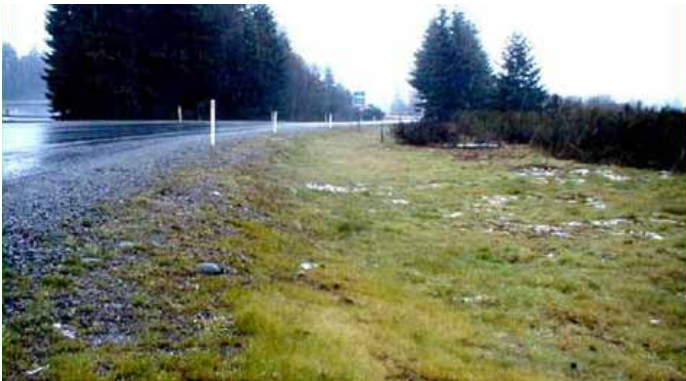
Natural dispersion areas like the one shown here provide a place for stormwater to infiltrate the ground or be taken up by the vegetation
