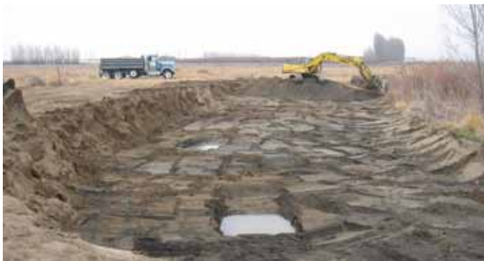
In November 2011, workers re-graded the U.S. 12 McNary Pond wetland mitigation site to produce more wetland area.
