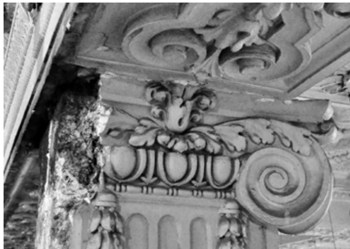
The project at Seattle's King Street Station restores the station's main hall as originally built in 1906 with white marble walls, decorative lighting and other features. This section of the ceiling has been covered for more than 50 years.
