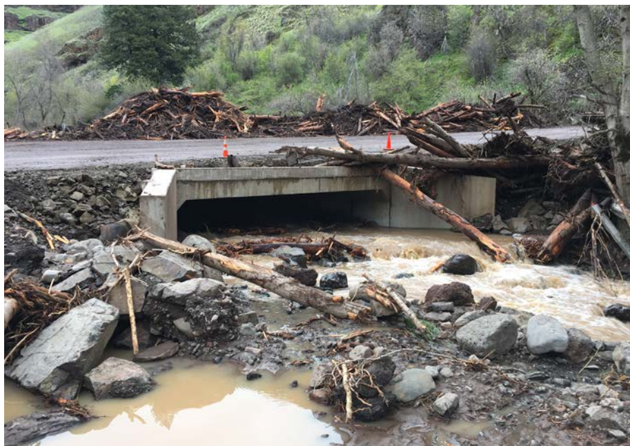
Above: Looking upstream at the corrected culvert of Rattlesnake Creek at SR 129 after the flood event of April 13, 2017. This fish passage barrier correction was completed in 2015 using a stream simulation culvert. Left: Rattlesnake Creek at SR 129 before WSDOT replaced the culvert that was creating a fish passage barrier.
