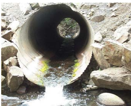
Above: Looking upstream at the corrected culvert of Rattlesnake Creek at SR 129 after the flood event of April 13, 2017. This fish passage barrier correction was completed in 2015 using a stream simulation culvert. Left: Rattlesnake Creek at SR 129 before WSDOT replaced the culvert that was creating a fish passage barrier.
