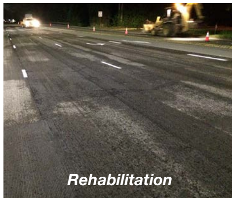
WSDOT crews repave a 1.5-mile stretch of SR 181 in Tukwila. This work costs about $250,000 per lane mile and will extend the life of the highway by an additional 14 years. It is substantially less costly than reconstructing the roadway.
