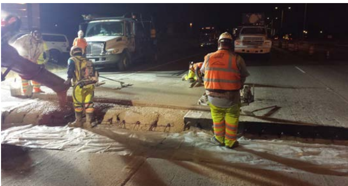
Contractor crews working for WSDOT replace 21 worn concrete panels on Interstate 5 between College Street in Lacey and 38th Street in Tacoma. Some of the concrete panels were installed when I-5 first opened during the early 1960s.
