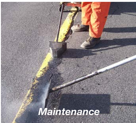
Crews perform crack sealing, a form of maintenance, along State Route 109. This is a relatively inexpensive treatment (about $5,000 per lane mile) that can extend the life of a roadway section by about three years.
