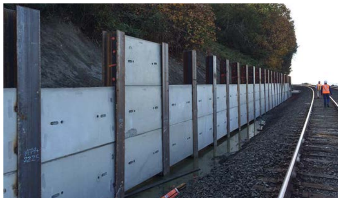
Retaining walls like the ones near Mukilteo being constructed in the photos above will catch landslide debris before it hits the tracks and will improve train reliability.
