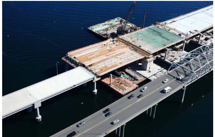
WSDOT crews construct the new SR 520 floating bridge's west end. The new bridge is set to open later this year. Tolling is on track to provide $1.2 billion for projects to improve safety and congestion on SR 520.
