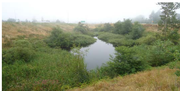
This stormwater basin has overgrown vegetation and does not adequately filter sediment from stormwater runoff. Approximately 19 percent of WSDOT's stormwater facilities are not yet in compliance.
