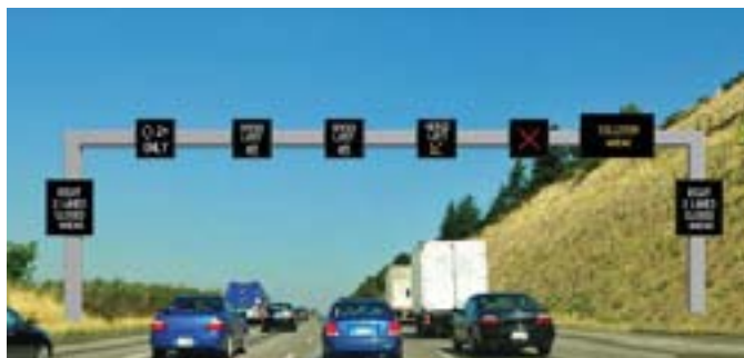
An artist's rendering of what a 'Smarter Highway' ITS system over I-5 might look like. Signs alert drivers to reduced speeds to maintain traffic flow and which lanes are blocked due to collisions. Visit www.smarterhighways.com for more information.
