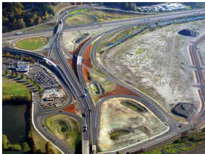
New ramps separate drivers and eliminate merges to help vehicles transfer smoothly and safely between I-5, SR 432 and Talley Way.
