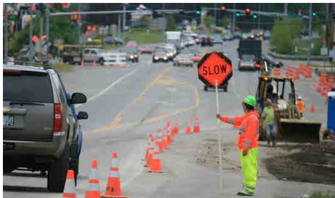
A flagger directs traffic during construction in 2010 to widen SR 410 and install a traffic signal at the intersection with 233rd Avenue East.
