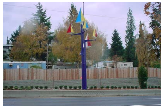
Exhibit V-1.4 – Urban Arterial with Median, Trees, and Low Profile Barrier (Location: SR 99, Des Moines, WA)
