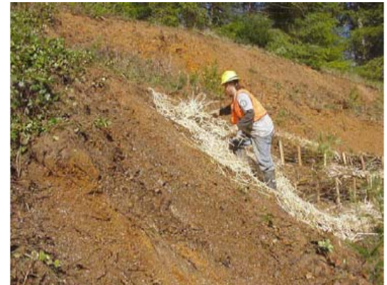
Exhibit IV-9.1 – Hand Distribution of Mulch (Recycled Woody Material) (Source: WSDOT Roadside Manual)
