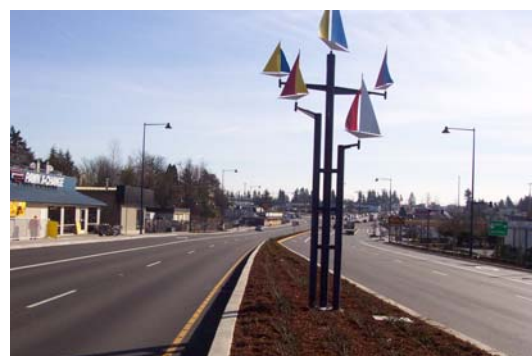
Exhibit A-1.14 – After Construction Southbound at 226 th
