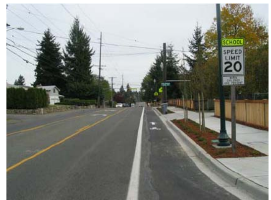
Exhibit III-1.2 – Pedestrian Facilities Provided Along a Roadway - Note the Buffer Zone and Speed Limit Sign (Location: Lacey, WA)
