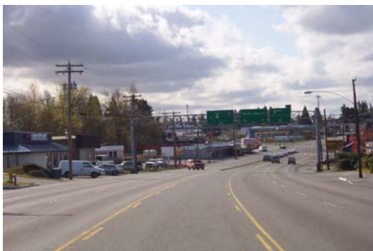
Exhibit A-1.13 – Before Construction Southbound at 226 th
