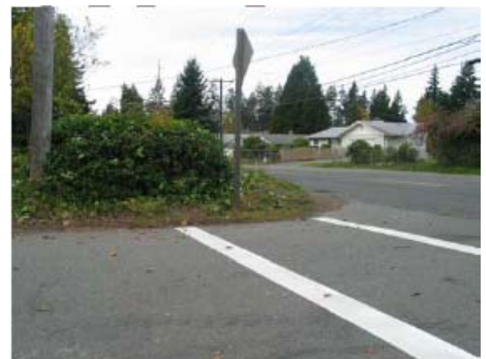
Exhibit V-5.13 – Lack of Intersection Sight Distance (Location: Pierce County, WA)
