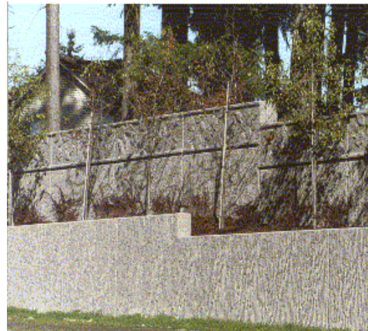
Exhibit A-2.6 – Top of Noise Wall Steps Mirrored with Retaining Wall
