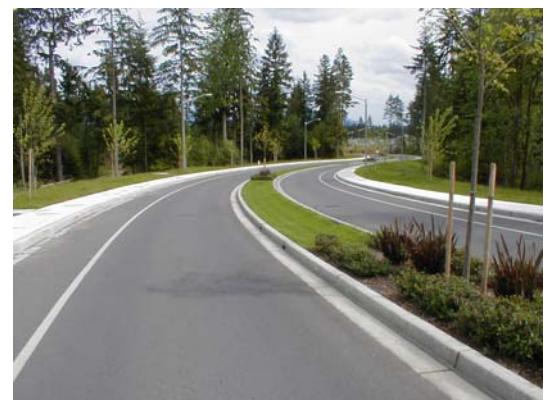
Exhibit III-2.2 – Shared Use Roadway (Location: Maple Valley, WA)
