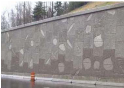
Exhibit IV-6.4 – Broad Leaf Pattern on Noise Wall (Location: Sunset Interchange on I-90, Issaquah, WA)
