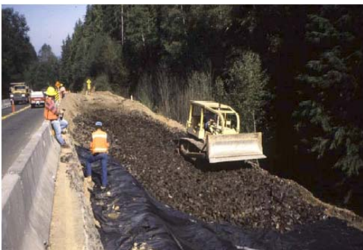
Exhibit IV-9.2 – Lightweight Tire Fill (Location: SR 101 South of Cosmopolis, WA)
