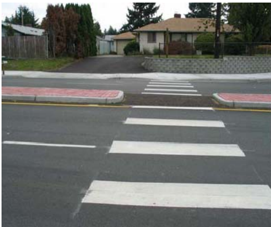
Exhibit III-1.16 – Marked Crosswalk with Median Refuge (Location: Lacey, WA)
