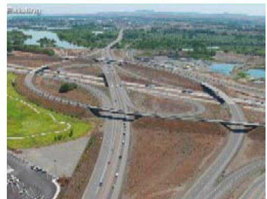
Exhibit A-7.3 – Existing Four Lanes
