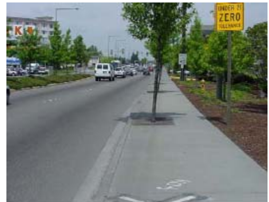
Exhibit V-11.3 – Vegetation Reducing Sign Visibility (Location: SR 99, SeaTac, WA)
