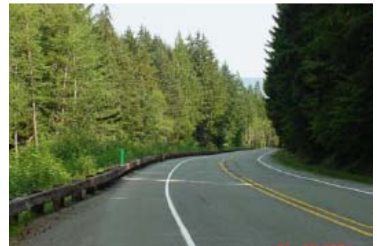
Exhibit V-4.9 – Guardrail System (Location: SR 410, Mather Memorial Highway, WA)
