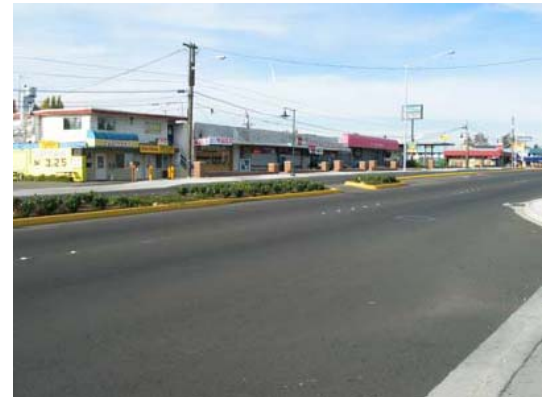
Exhibit III-1.19 – Unmarked Mid-block Pedestrian Crossing with Median Refuge (Location: Tukwila, WA)
