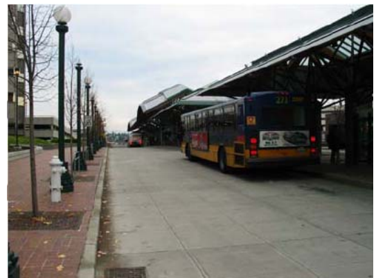
Exhibit III-1-26 – A Transit Facility (Location: Bellevue, WA)
