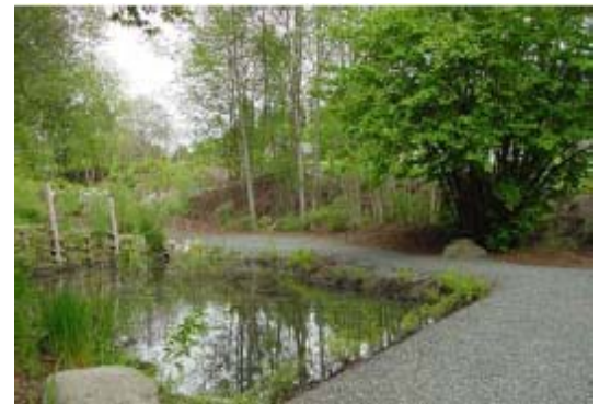
Exhibit V-13.1 – Indian Creek Stormwater Facility (Location: Olympia, WA)
