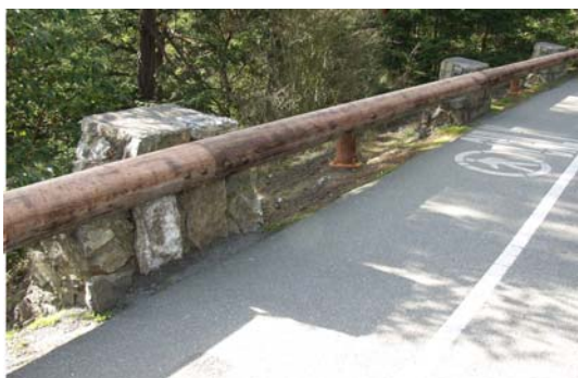
Exhibit IV-4.5 – Retrofitted Rail Using Historic Features (meets current day design requirements) (Location: Deception Pass, WA)
