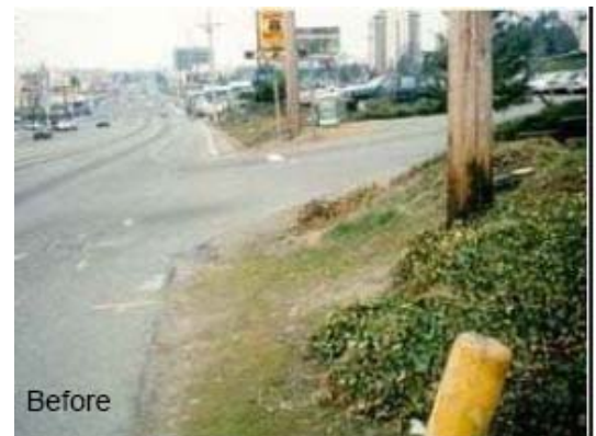
Exhibit V-6.4 – Access Before and After Streetscape Redevelopment (Location: SR 99, SeaTac, WA)
