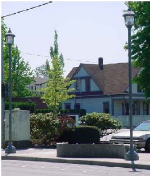
Exhibit V-10.2 – Additional Illumination Fixtures (Location: Kent, WA)
