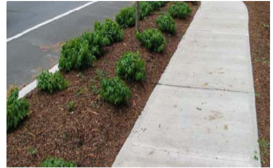
Exhibit III-1.18 – Buffer Zone Provided Between the Roadway and a Sidewalk (Location: Sammamish, WA)
