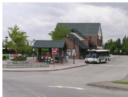
Exhibit III-3.7 – Off-Street Transit Center (Location: Vancouver, WA)
