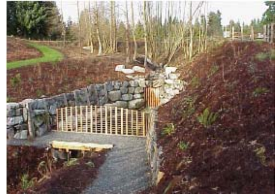
Exhibit VI-3.4 – Indian Creek Stormwater Facility (Location: Olympia, WA)
