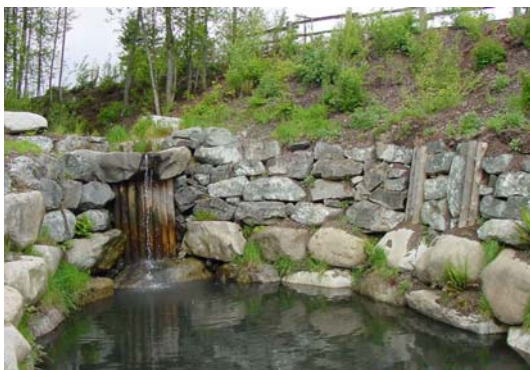
Exhibit IV-2.2 – Stormwater Facility (Location: Indian Creek, Olympia, WA)
