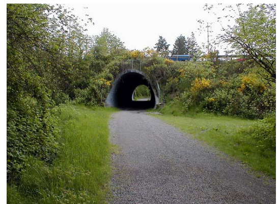
Exhibit III-2.6 – Lake Wilderness Trail Underpass (Location: Maple Valley, WA)
