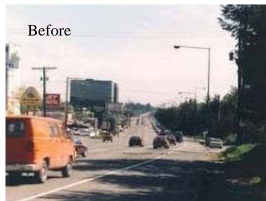
Exhibit V-6.6 – Streetscape Before and After Turning Movement Definition (Location: SR 99, SeaTac, WA)
