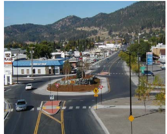
Exhibit A-4.5 – Finished Roundabout
