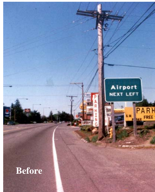
Exhibit V-7.3 – Utility Undergrounding (Location: SR 99, SeaTac, WA)
