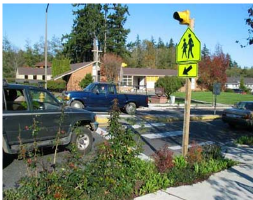
Figure III-1.24 – A Flashing Beacon to Improve Visibility of the School Zone Pedestrian Crossing (Location: Bainbridge Island, WA)
