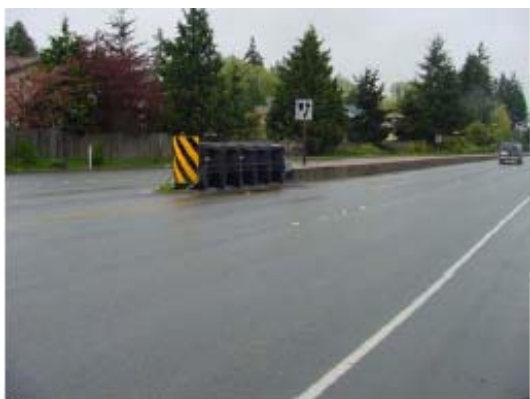
Exhibit V-4.12 – Impact Attenuator Protecting the End of a Low Profile Barrier (Location: SR 303, Bremerton, WA)
