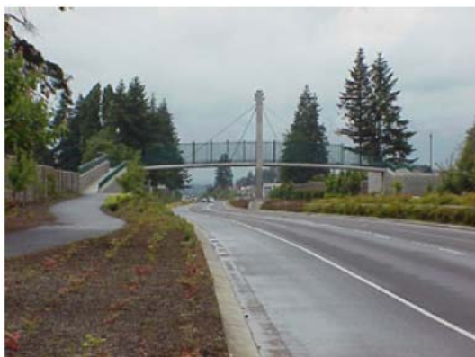
Exhibit V-1.3 – Pedestrian Overpass (Location: Clark County, WA)
