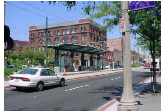
Exhibit II-2.7 – Multi-Modal Facility (Location: Tacoma, WA)
