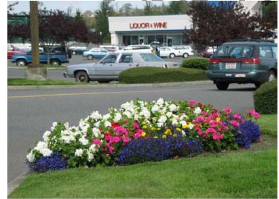
Exhibit III-1.11 –Landscaping at an Intersection that Facilitates Pedestrian Visibility (Location: Sequim, WA)
