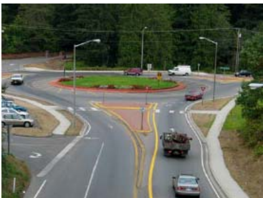
Exhibit V-5.10 – Center Islands With and Without Landscaping (Locations: Bethel Ave/SR 166/Mile Hill Drive and SR 203/Novelty Hill Road, Duvall, WA)
