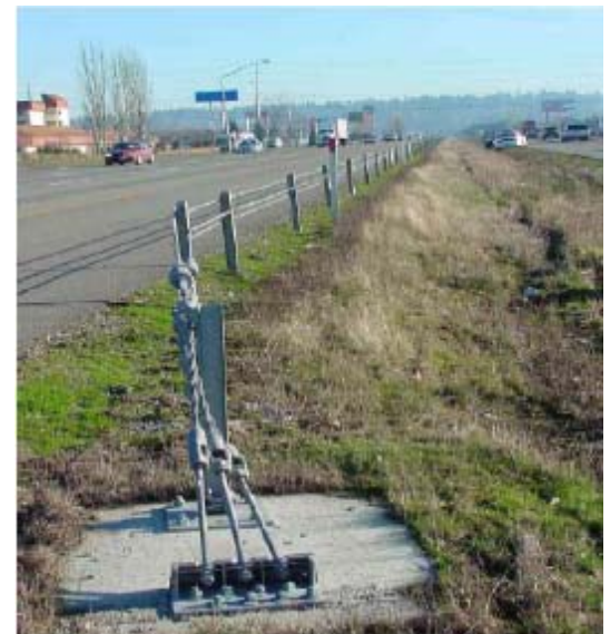
Exhibit V-4.10 – Cable Median Barrier (Location: I-5, Tacoma, WA)
