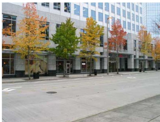
Exhibit III-1.25 – Streetscape Amenities and Trees Along a Roadway (Location: Bellevue, WA)
