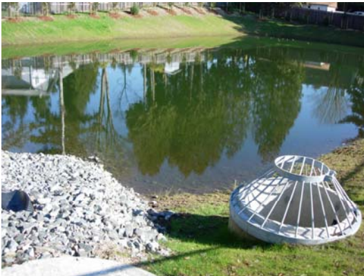
Exhibit A-1.8 – Stormwater Facility
