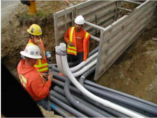
Exhibit A-1.7 – Undergrounding Utilities
