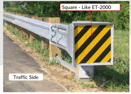
Some SKT Terminals still have a ground strut and wood posts. If the terminal has a ground strut and steel posts, it is an MSKT and NOT an SKT.
