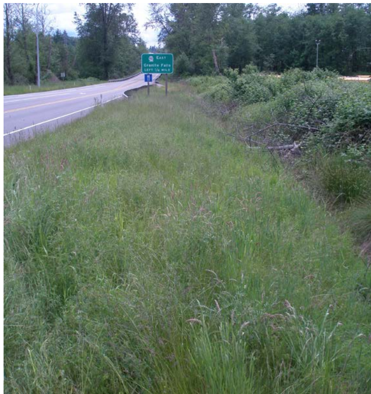
Figure 2 VFS on the shoulder embankment of State Route 9 near Marysville, WA.
