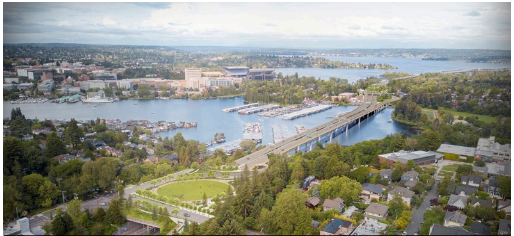
Renderings superimposed on drone images became important tools to help share the community vision of the extensive SR 520 Project
