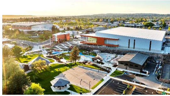
Completed Riverfront Park North Bank Playground
