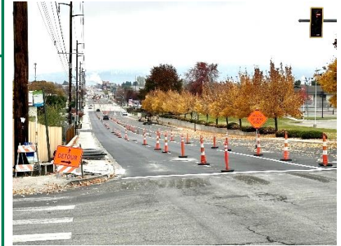
Preservation and enhancement work underway
