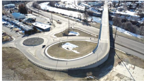
Completed bridge replacement
