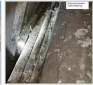
Pier 18's bearing is compressed, which means that the bridge cannot move as it should. Instead, the bearing is creating additional pressure on the surrounding area and affecting the bridge as a whole.
