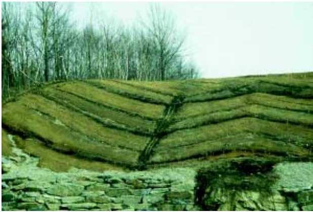
Live facine installation-angled. Robbin Sotir & Associates
