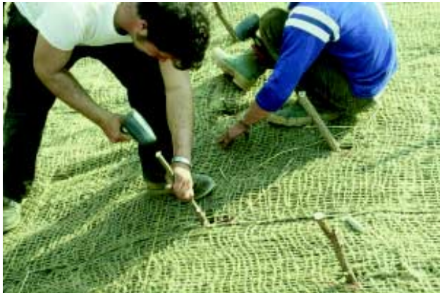
Live staking. Robbin Sotir & Associates
