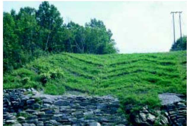
Live facine installation-angled. Robbin Sotir & Associates
