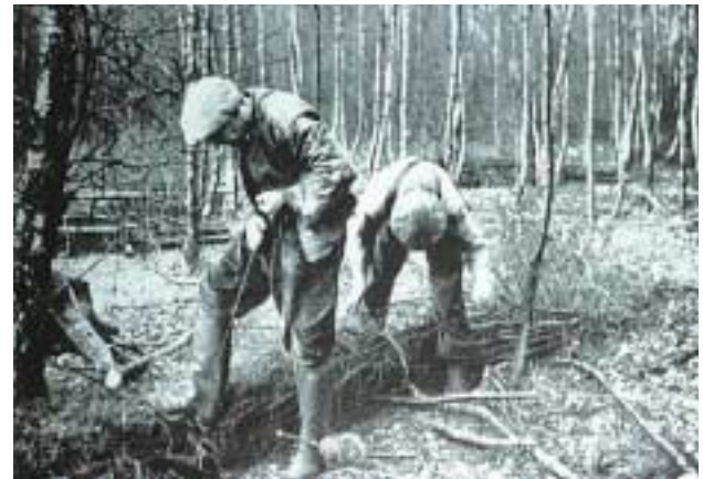
Europe Early 1900's. Cutting and collection of live stems for soil bioengineering. Kevin Finney
