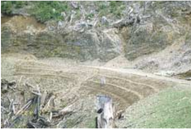
Hand excavated terraces for erosion control blanket. USDA Forest Service
