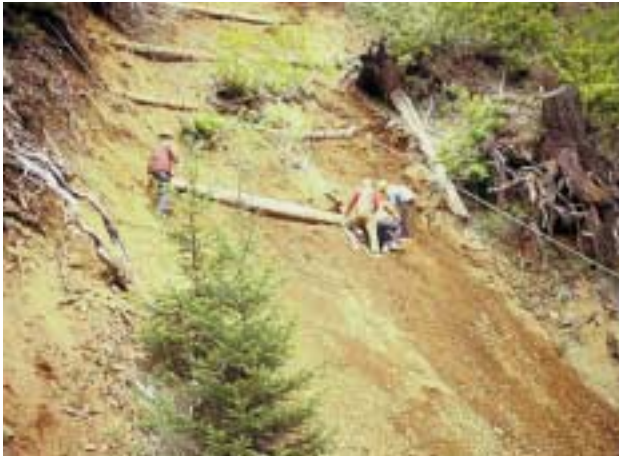
Installation - cutslope stabilization with log terracing. USDA Forest Service
