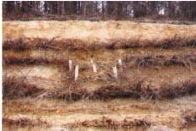
Branchpacking just after installation. Robbin Sotir & Associates
