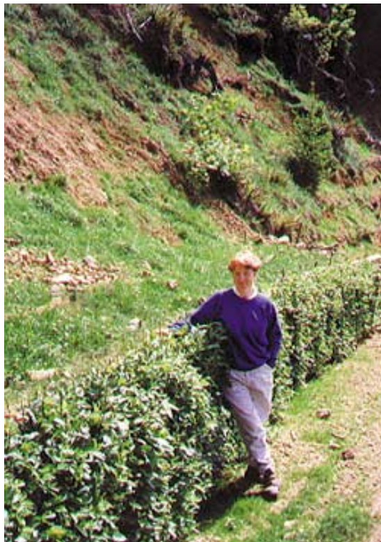
Live cribwall one month after construction. USDA Forest Service
