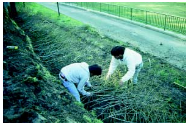
Brushlayer installation. Robbin Sotir & Associates
