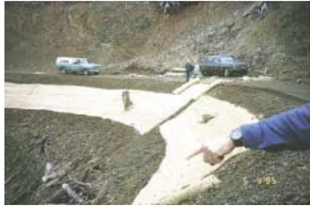
Rolling out erosion control blanket. USDA Forest Service
