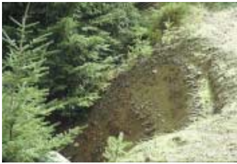
Brushlayering just after installation. Robbin Sotir & Associates
