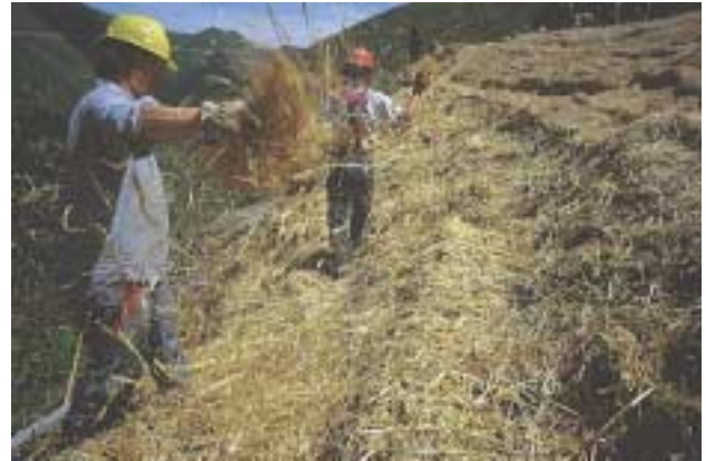
Spreading straw mulch. USDA Forest Service
