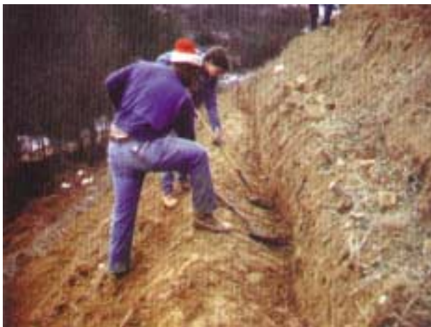
Digging terraces for brushlayer installation. Robbin Sotir & Associates.
