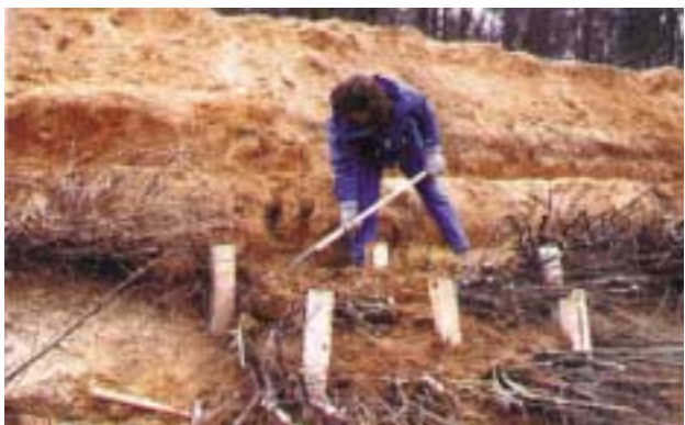
Branchpacking just after installation. Robbin Sotir & Associates
