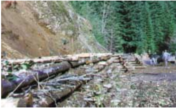
Live cribwall during construction. USDA Forest Service
