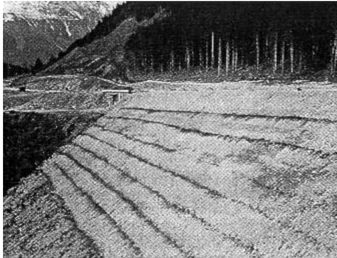
Figure 6. Brushlayer embankment fill stabilization immediately after construction Brenner Pass highway, Austria.
