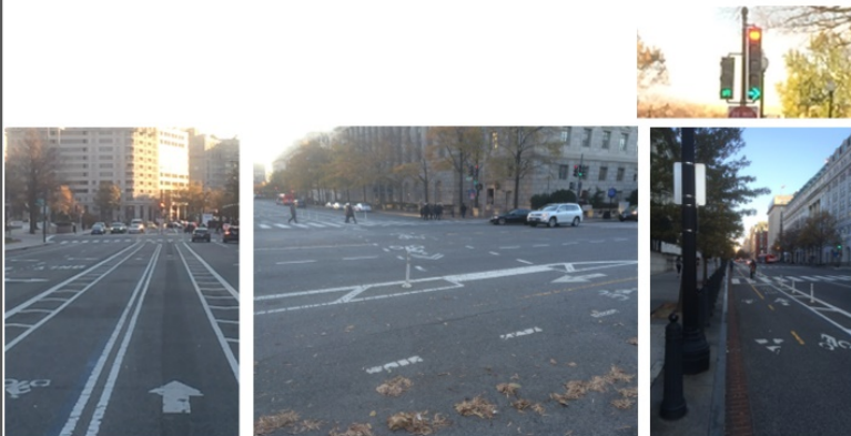
Two-way Cycle Tracks, Pennsylvania Ave NW and 15 th Street NW, Washington D.C.
