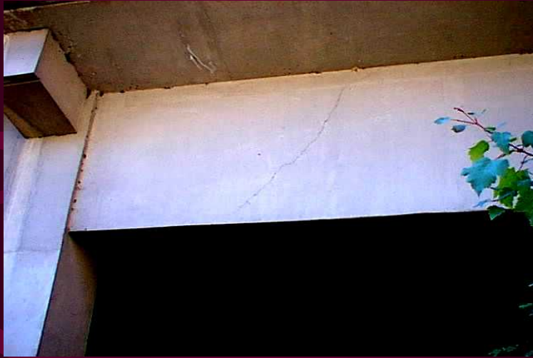
BR 08429E Grande Ronde River, Quarry Bridge
