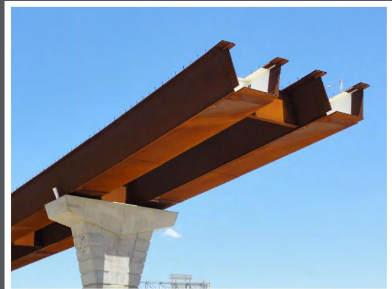
Figure 12.1 Dual Steel Trapezoidal Box Girders
