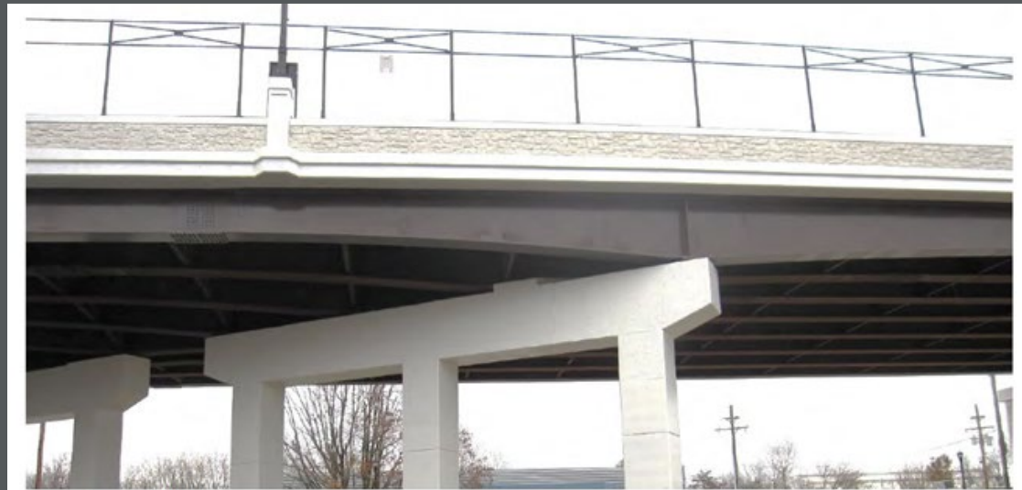
Figure 10.25 Application of Parabolic Variable Depth Girders
