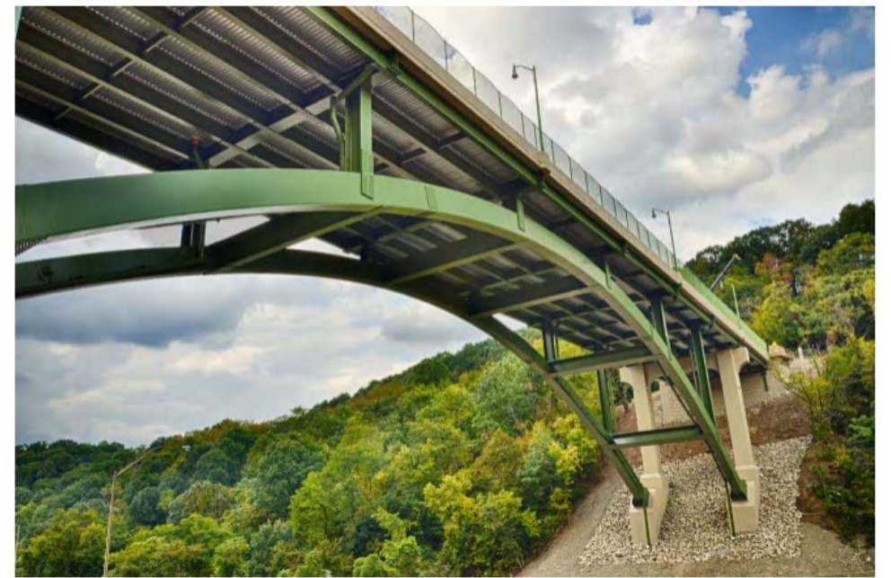
Figure 14.1 Greenfield Bridge in the City of Pittsburgh, an Open-Spandrel Deck Arch Structure Completed in 2017
