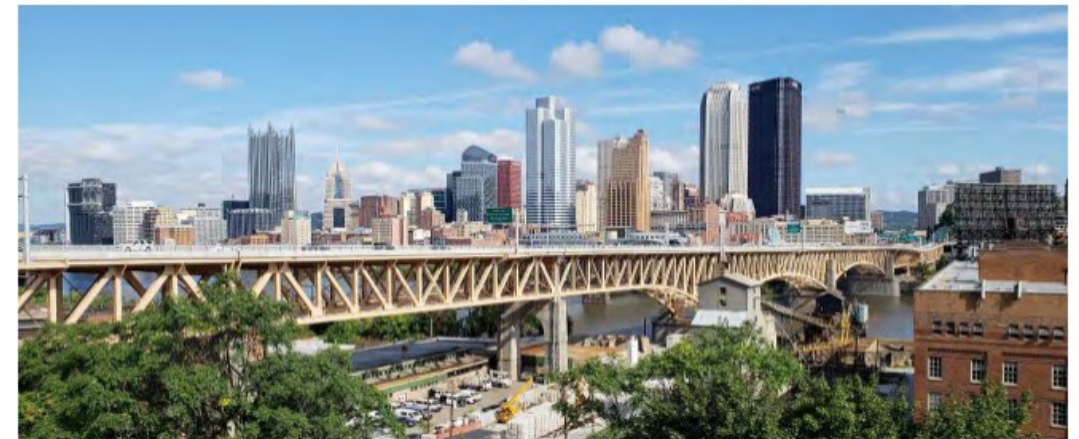
Figure 13.4 Deck Truss Bridge, Liberty Bridge over the Monongahela River in Pittsburgh, Pennsylvania
