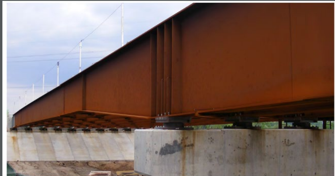
Figure 10.26 Application of Straight Taper Variable Depth Girders
